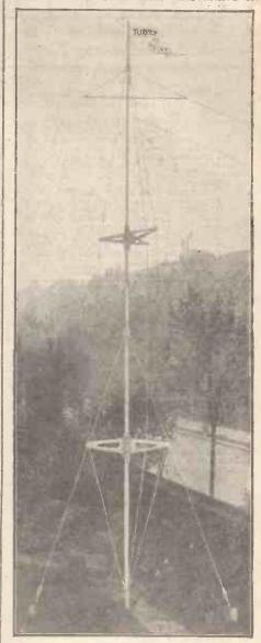
Photo of the Patent Turret Oregan Pine Cantilever Magt designed by Naval Experts.
