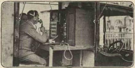
This mobile wireless telephony installation was fitted on a motor-van by the Marconi Company. A power of 500 watts is employed, and excellent results have been obtained. Our illustration shows an operator speaking from Epsom to Marconi House,
