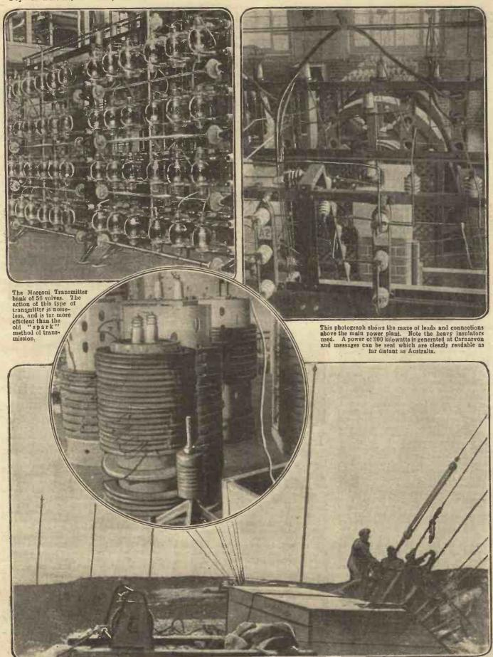
Our photograph in the circle above shows the choke coils used in connection with the old "spark" transmitter. Below, the photograph shows some of the ten steel masts, each 400 feet high, which support the aerial system. The gny ropes are anchored to massive 100-ton concrete blocks and are capable of withstanding an enormous strain.
