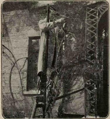
The insulation of the lead in wire is very important indeed. A fault at the lead in tube means a "Short" to earth, and consequently your received signals will he dead weak, if any get through at all.
