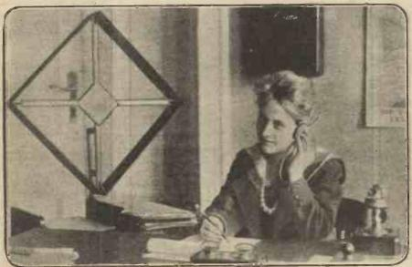
The advantages of a frame aerial will be seen in this picture. No be easily mounted on a desk, No outside wire is necessary, and it can
