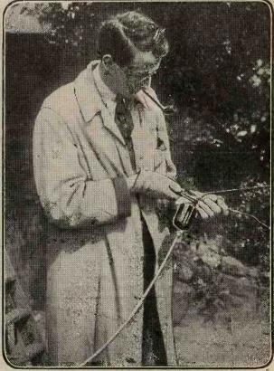
Attach the Aerial securely to the insulators. When the aerial is aloft it will have to take a big strain, and a bad connection will mean a collapsed aerial when you wake up one fine morning.
