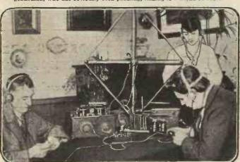
Wireless in the drawing-room without an aerial! Our photograph shows a wireless set which requires no outside wires. The frame aerial shown, when used in conjunction with valve amplifiers, picks up excellent signals from the Eiffel Tower and many other wireless stations,
