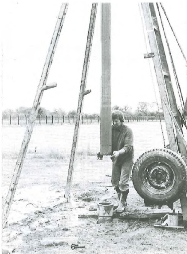
FIG. 4—Site investigation rig showing cutting tool and top of borehole lining tube
