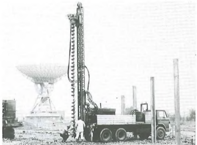
FIG. 8—Augering through the gravel layer prior to pile driving
