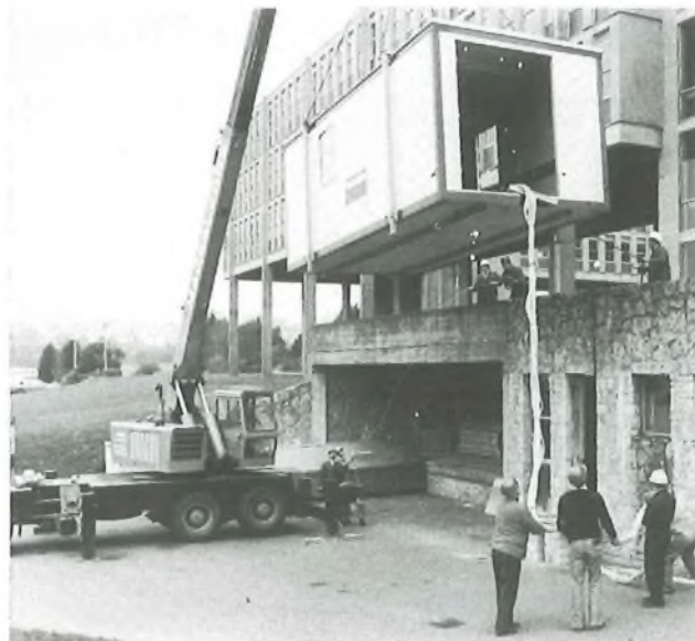
FIG. 3—The Portakabin being hoisted into position
