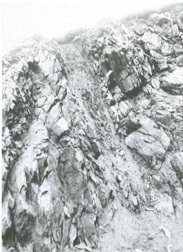
FIG. 3—Shetland: clay-filled fault about 1 m wide
