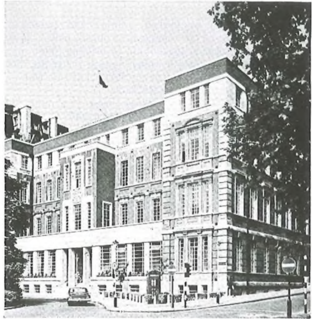
FIG. 2—The IEE building, Savoy Place, London
