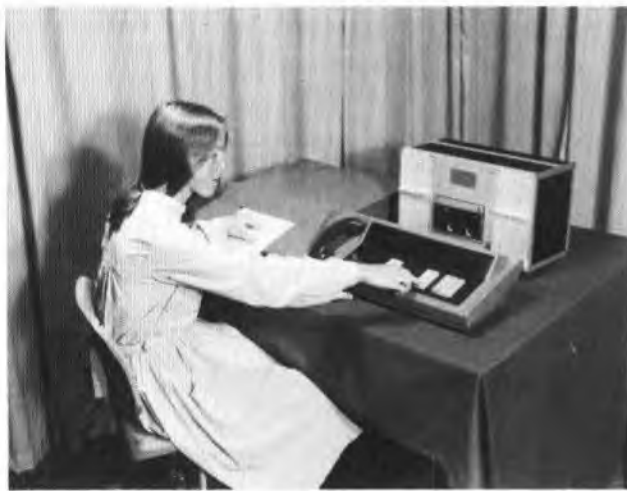
FIG. 2—Document being loaded into the Fonofax SF system
