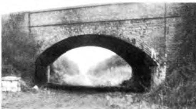
FIG. 1—The bridge before demolition, viewed from the level of the old railway track
