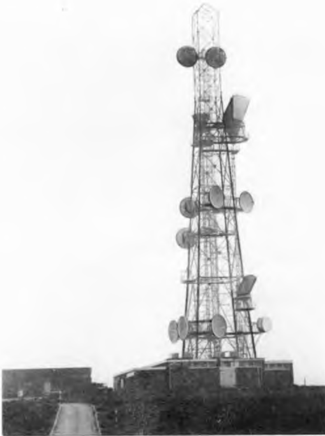
Fig. 30—Typical BPO radio station
