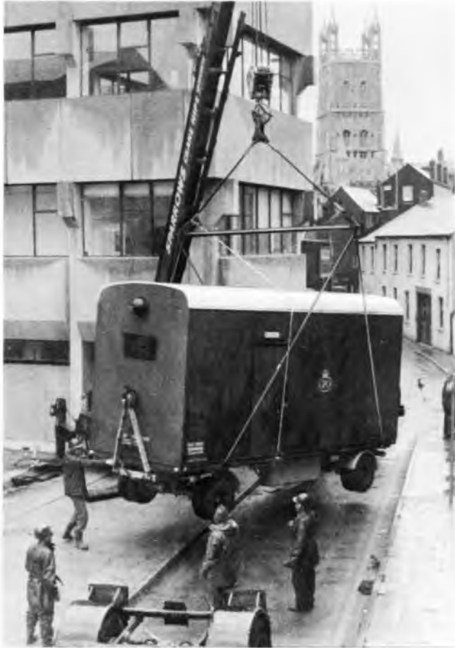
FIG. 3—Mobile unit 7 being removed from the compound
