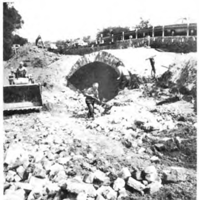
FIG. 3—Demolition of the bridge, with masonry being deposited on the new duct line
