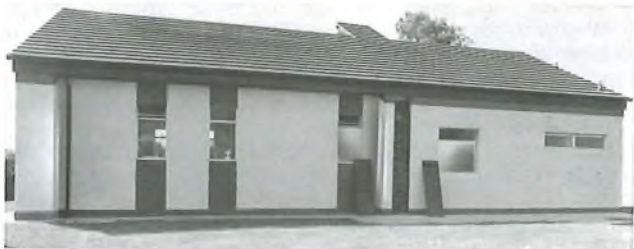
General view of Q-type building, showing vertical riser (centre)
