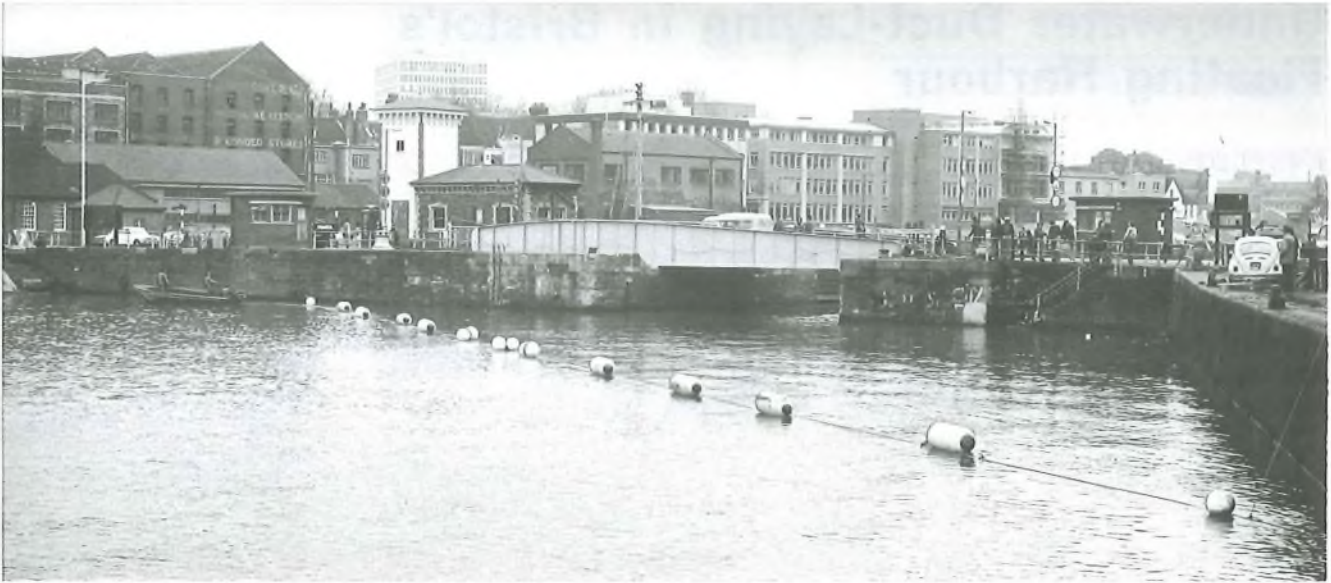
FIG. 3—Towing the ducts into position across the harbour
