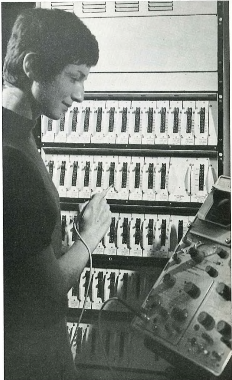
Marconidata multiplex/demultiplex equipment
