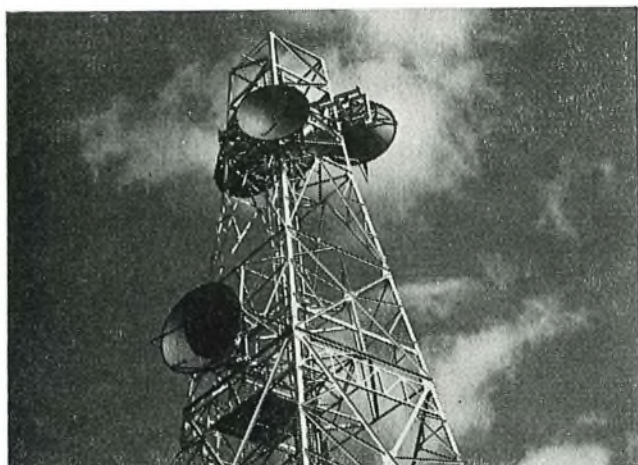
A typical antenna tower installation.
