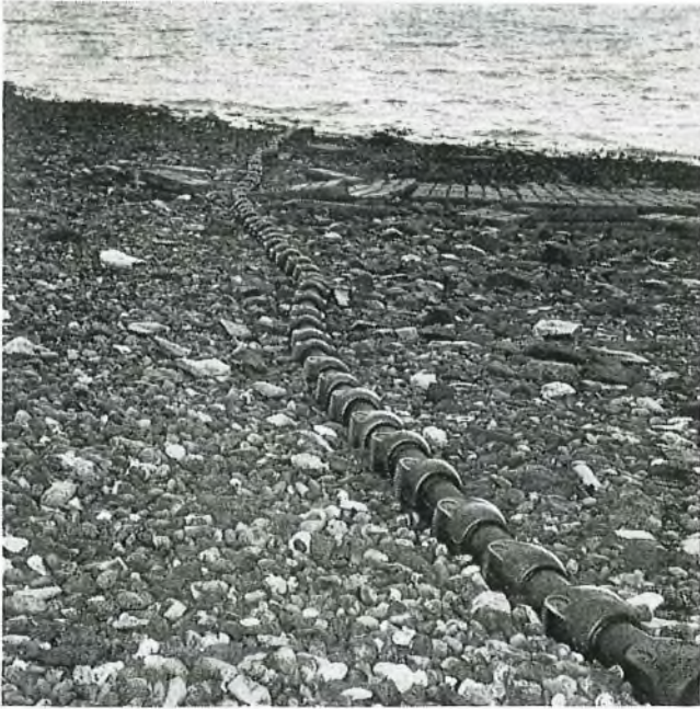
FIG. 1—Cast-iron split-ducts fitted to cable
