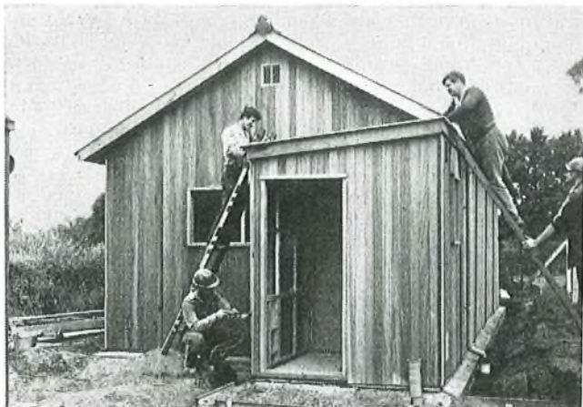
Erection of Silverton S.A.X.
