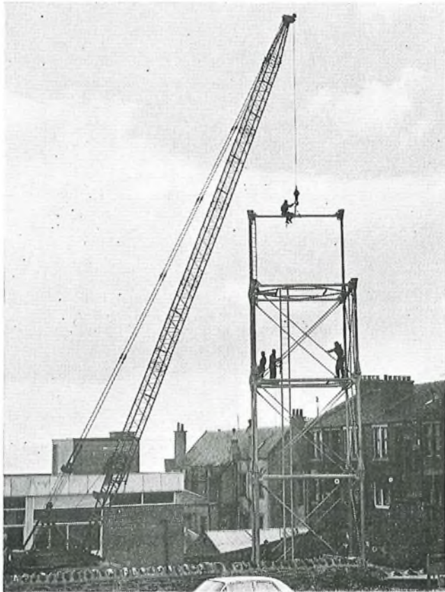
FIG. 1—Mobile crane being used to erect the radio tower.
