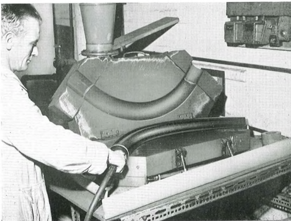
FIG. 3—Mould for production of bends
