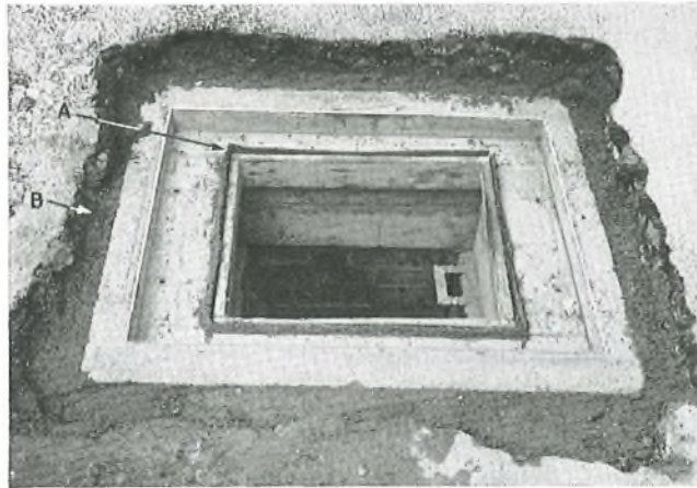
A—Rubber shuttering B—Dry concrete backfill
