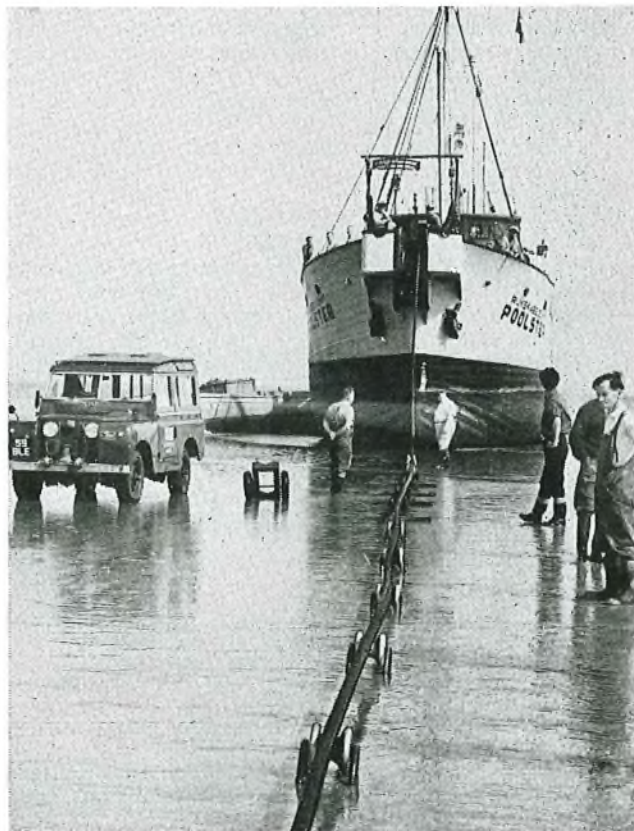
CABLE BEING HAULED ASHORE FROM POOLSTER
