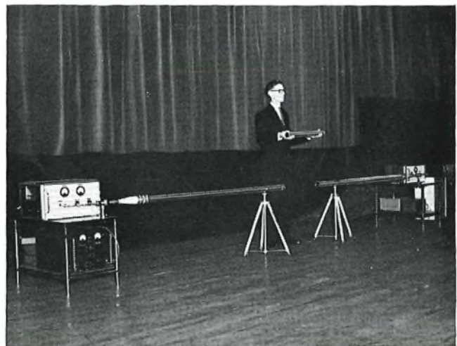
FIG. 7—DEMONSTRATION OF THE WAVEGUIDE
