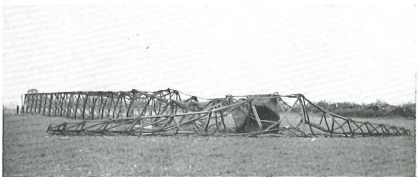
FIG. 2—MAST AFTER BEING FELLED
