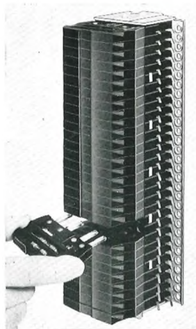
FIG. 1.—FUSE UNIT USED AT SPRINGPARK EXCHANGE
