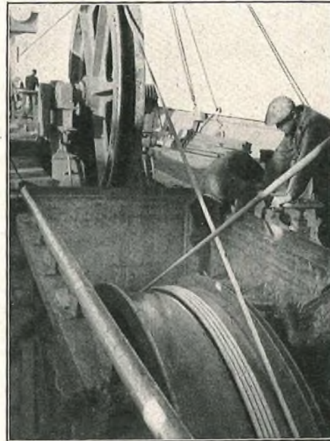
FIG. 1.—RECOVERY OF THE FIRST LIGHT-WEIGHT CABLE FROM 2,600 FATHOMS (3.1 MILES).
