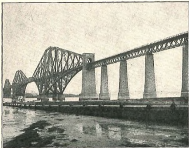
FIG. 1.—GENERAL VIEW OF BRIDGE AND SOUTHERN APPROACH.
