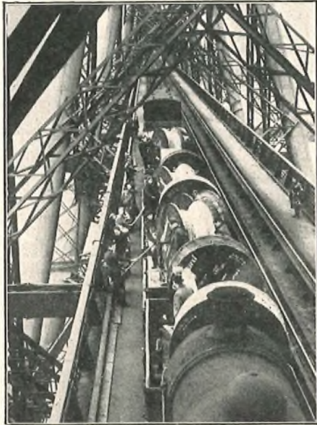
FIG. 11.—CABLING ACROSS BRIDGE FROM TRAIN.
