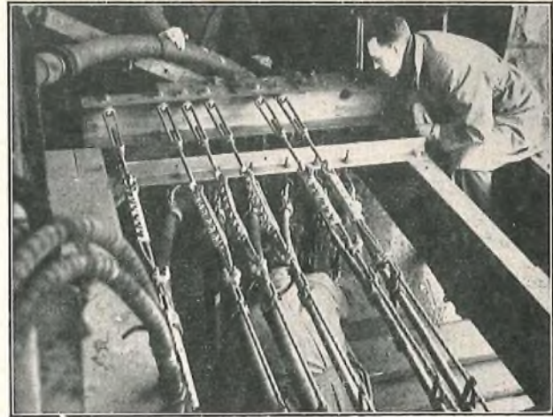
FIG. 5.—TERMINATION OF CABLE SUSPENSION WIRES.
