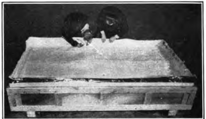
FIG. 4.—SEALING MOISTURE VAPOUR BARRIER LID IN POSITION.
