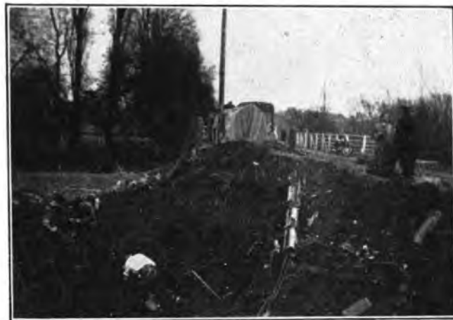
CABLE REPAIRS IN PROGRESS.
