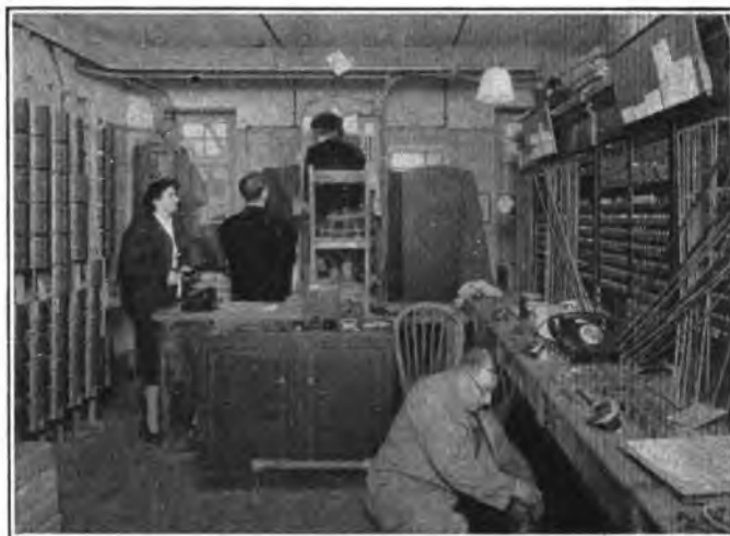
P.B.X. 10 + 50 MOUNTED ON PLATFORM IN CANVEY EXCHANGE.
