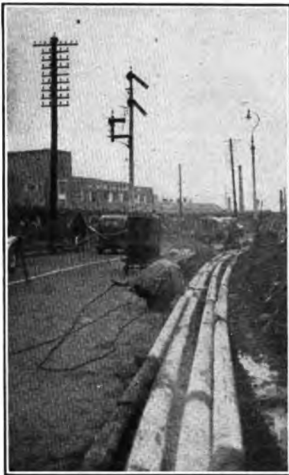
THE DIVERSION IN PROGRESS.
