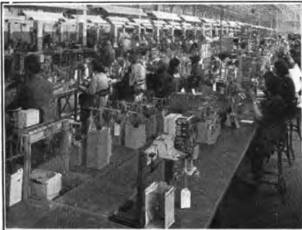
ASSEMBLY AND WIRING SHOP.
