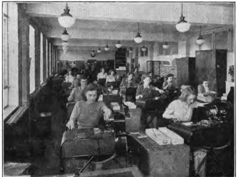
FIG. 4. THE CANTERBURY INSTALLATION.
