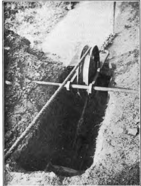
CABLING AID IN USE FOR DIRECT PULL—SPLIT COUPLING.
