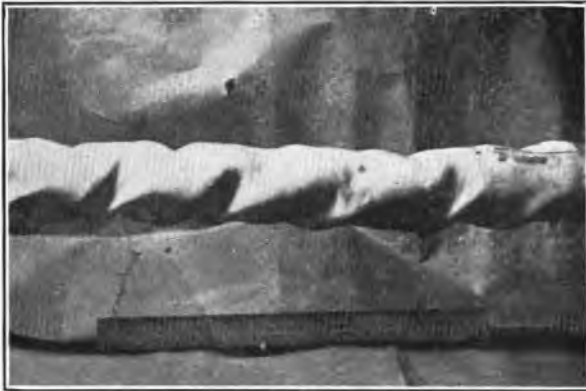
DAMAGE TO CARMARTHEN-MILFORD HAVEN AERIAL CABLE.
