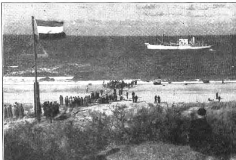
FIG. 4.—H.M.T.S. Alert LAYING SHORE END AT DOMBURG.
