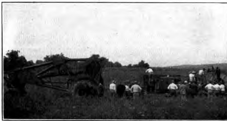
FIG. 2.—LAYING A COAXIAL CABLE BY GIANT PLOUGH.
