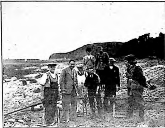
FIG. 2.—STATES TELEPHONE DEPARTMENT JOINTER WORKING UNDER ESCORT ON SUBMARINE CABLE AT FLIQUET.
