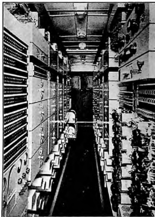
FIG. 5.—D.T.N. MOBILE TELEGRAPH TERMINAL (VIEWED FROM FRONT).
