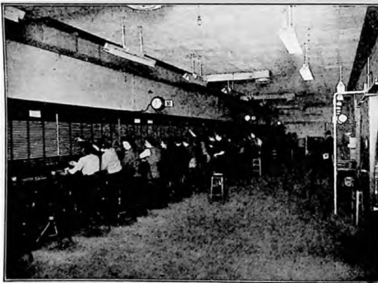
FIG. 2.—CITADEL TRUNK SWITCHBOARD.
