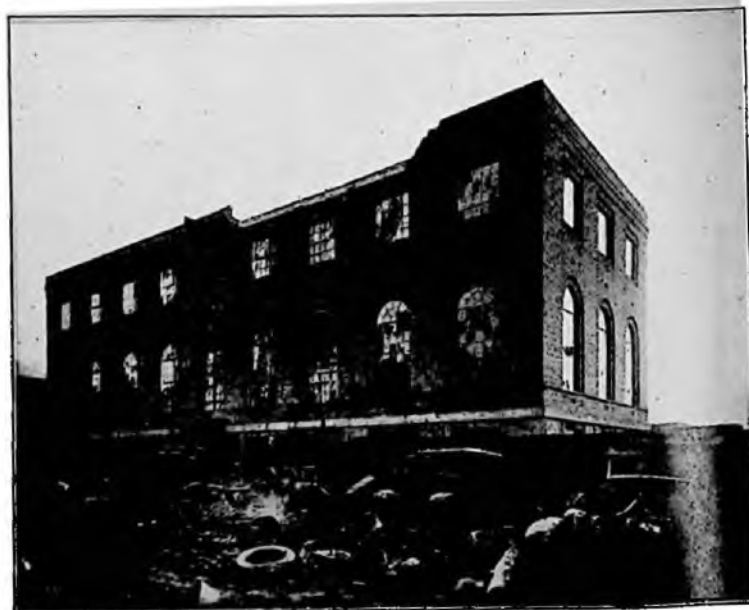
FIG. 3.—DAMAGE TO AN AUTOMATIC EXCHANGE (VICTORIA EXCHANGE, BIRMINGHAM).
