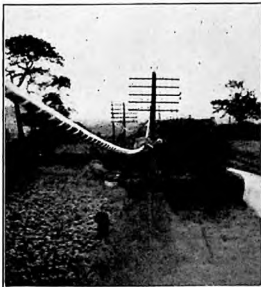
FIG. 4. CABLE SPAN PARTLY COMPLETED.
