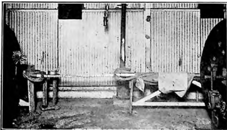
FIG. 3.—" UNIDIAMETER " JOINT PARTIALLY COMPLETED.
