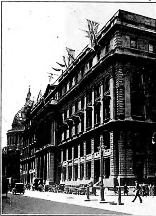
Fig. 1.—C.T.O. BUILDING IN 1935.
