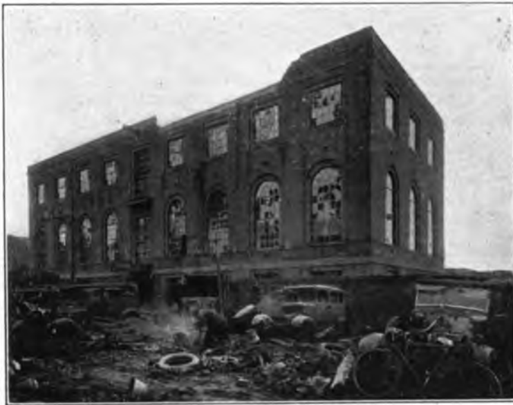
FIG. 2.—EFFECT OF BLAST ON A PROVINCIAL TELEPHONE EXCHANGE BUILDING.
