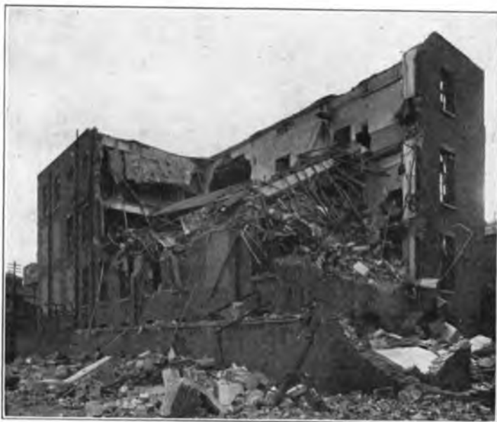
FIG. 1.—COMPLETE DESTRUCTION OF A LONDON TELEPHONE EXCHANGE BUILDING.
