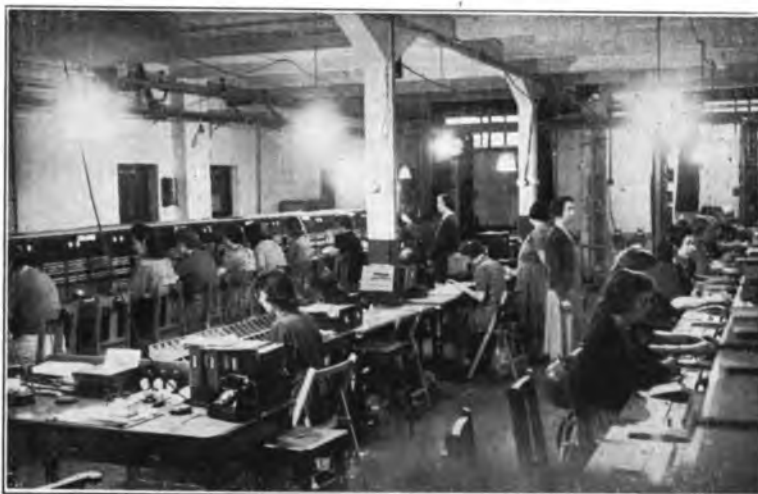
FIG. 6.—A TYPICAL EMERGENCY EXCHANGE.
