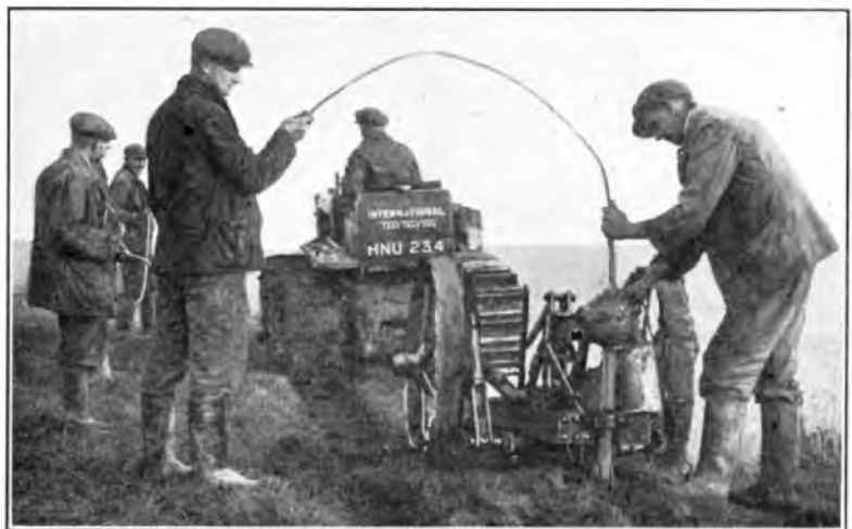
FIG. 2.—CABLE-LAYING WITH MOLEDRAINER.
