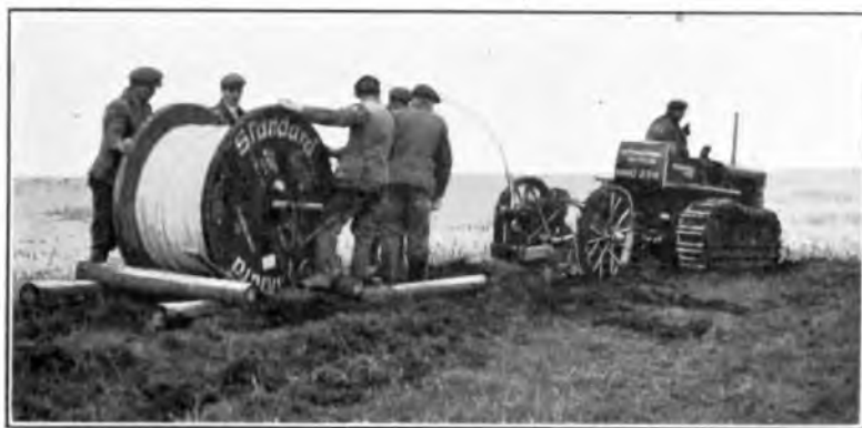
FIG. 3.—CABLE-LAYING WITH MOLEDRAINER AND SLEDGE.
