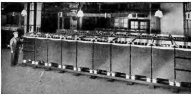
Two batteries of Alton Cells at Blackfriars Telephone Exchange, Manchester.
