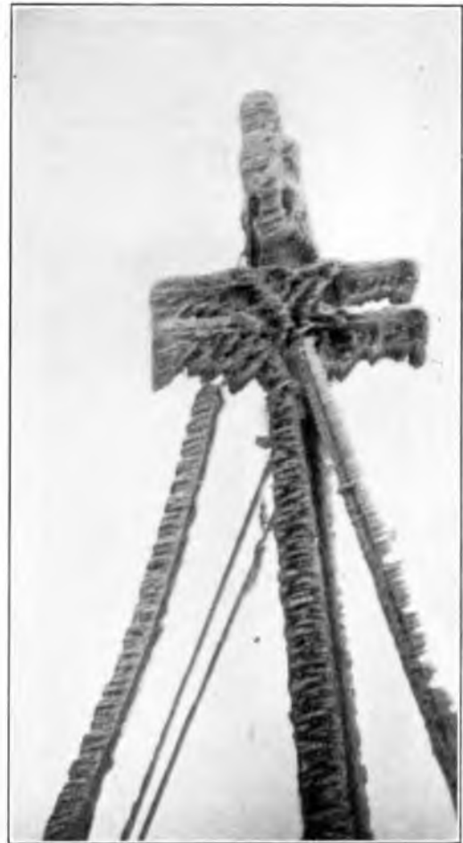
FIG. 4.—POLE HEAD ENCASED IN ICE.
