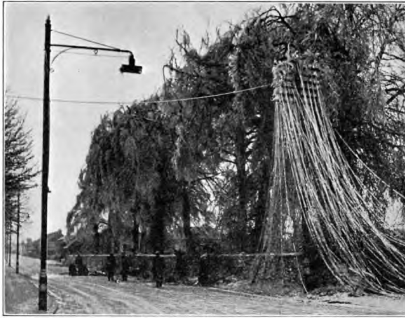
FIG. 7.—DAMAGE IN THE BRISTOL AREA.
