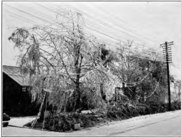
FIG. 11.—FALLEN WIRES ON THE SOUTHAMPTON-WINCHESTER ROUTE.
