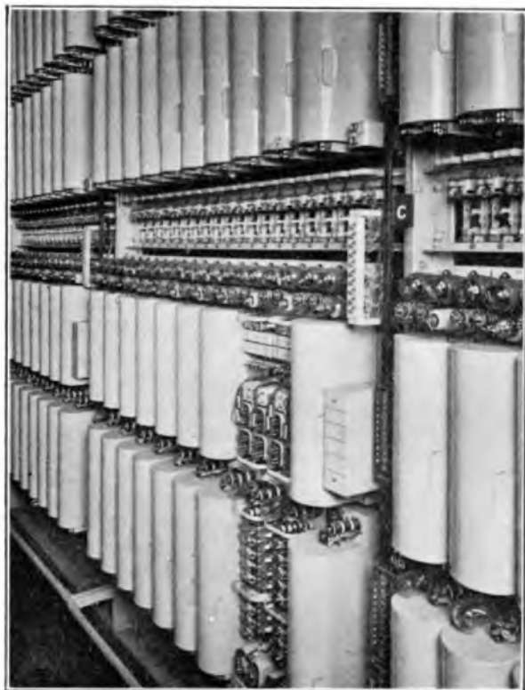
FIG. 7.—O.G. AUTO RELAY SETS AND 2 V.F. RECEIVERS.
