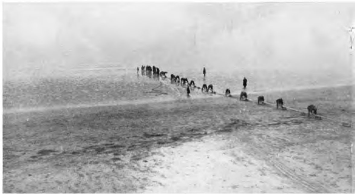
LAYING SUBMARINE TELEPHONE
