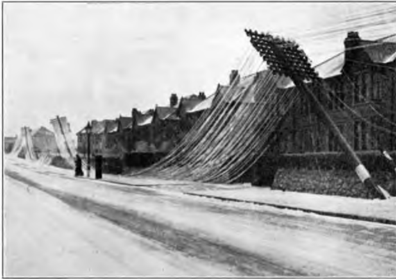
FIG. 3.—DEFLECTED POLES AT CYNCOED, CARDIFF.
