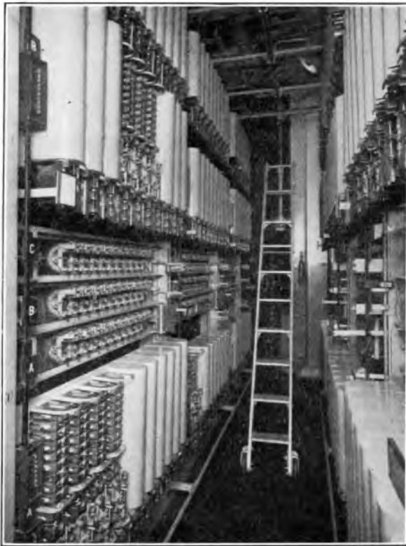
FIG. 5.—TRUNK 1ST CODE SELECTORS.
