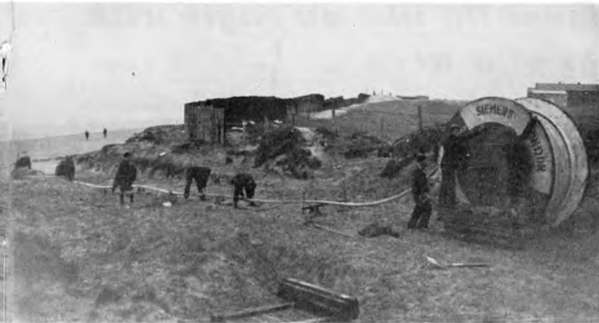
NE CABLE ACROSS AN ESTUARY
