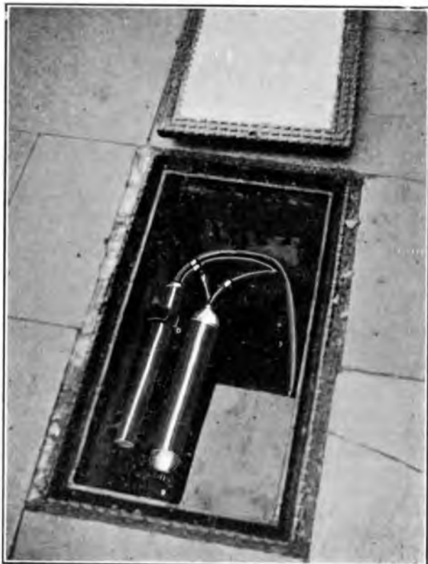
FIG. 3.—AUXILIARY JOINT IN FOOTWAY JOINTING CHAMBER.
