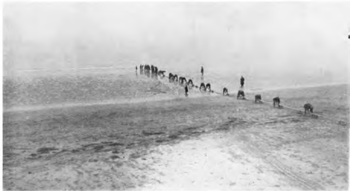
LAYING SUBMARINE TELEPHONE CABLES
