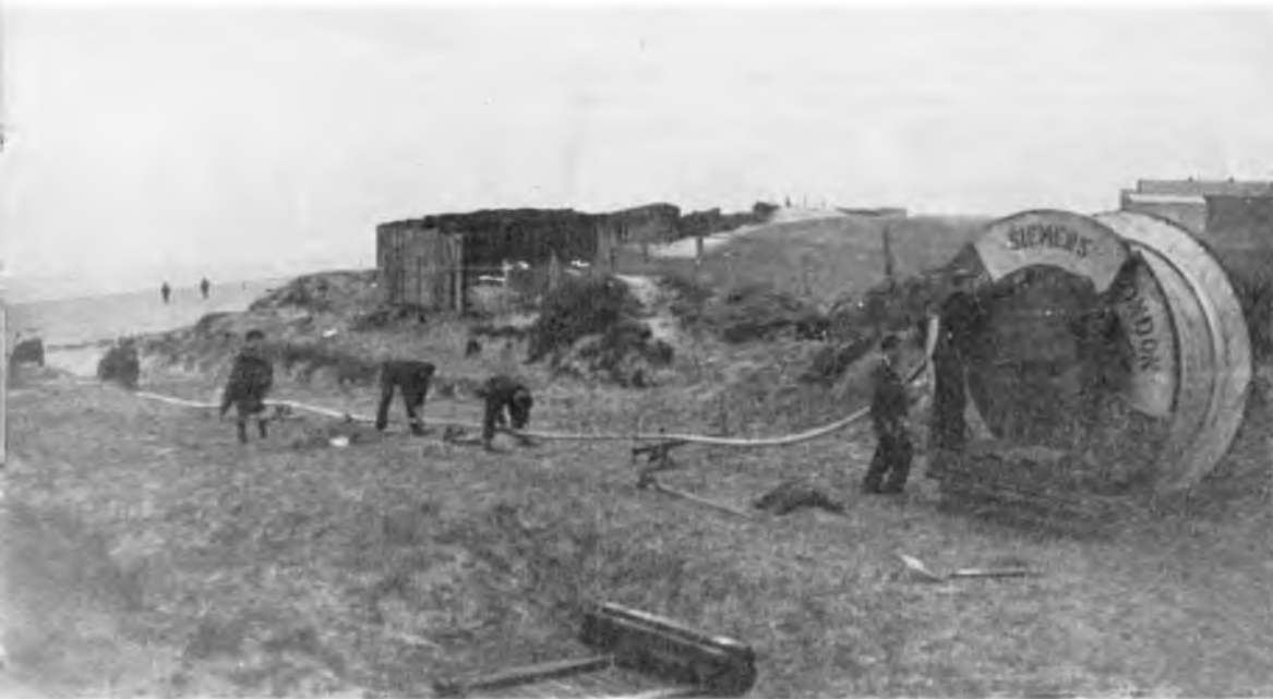
E CABLE ACROSS AN ESTUARY
