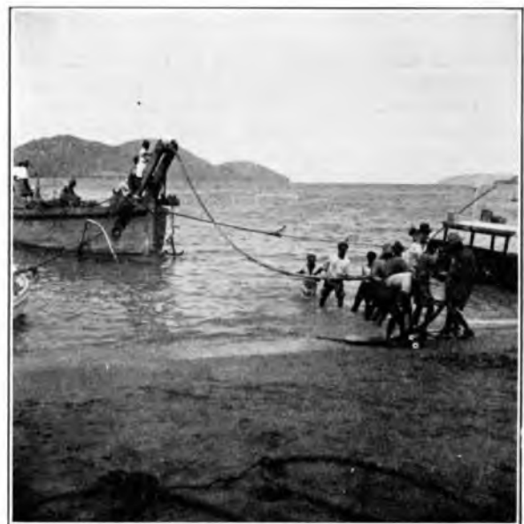
FIG. 8.—LANDING THE SHORE-END.
