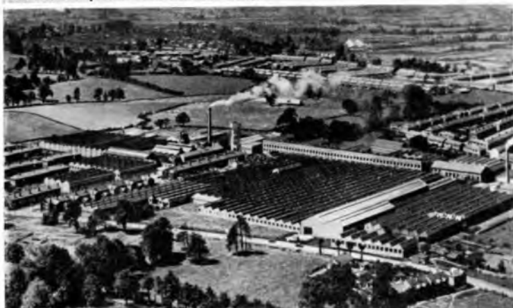
G.E.C. Telephone Works, Coventry
