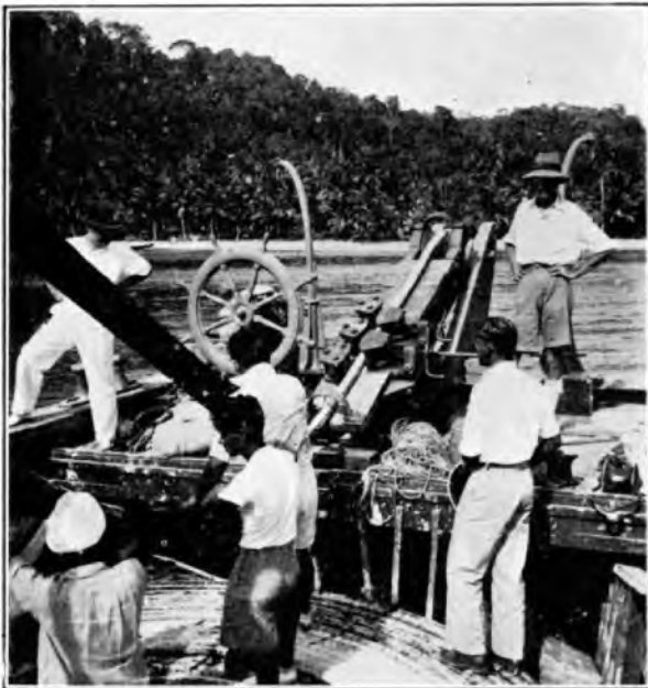
FIG. 6.—VIEW OF CABLE BRAKE AND STERN OF LIGHTER.
