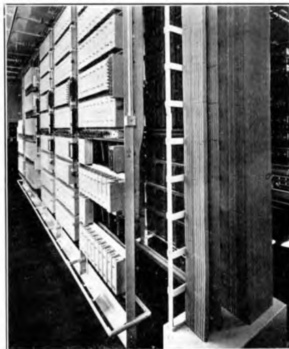
FIG. 7.—SUBSCRIBERS' L AND K RELAY RACKS.
