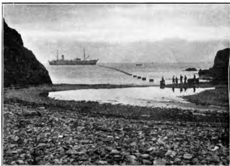
FIG. 5.—LANDING CABLE DIRECT FROM C.S. FARADAY AT ABERGEIRCH.
