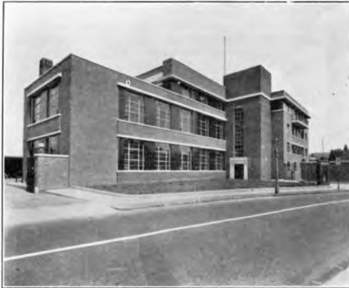
FIG. 1.—KINGSTON EXCHANGE BUILDING.
