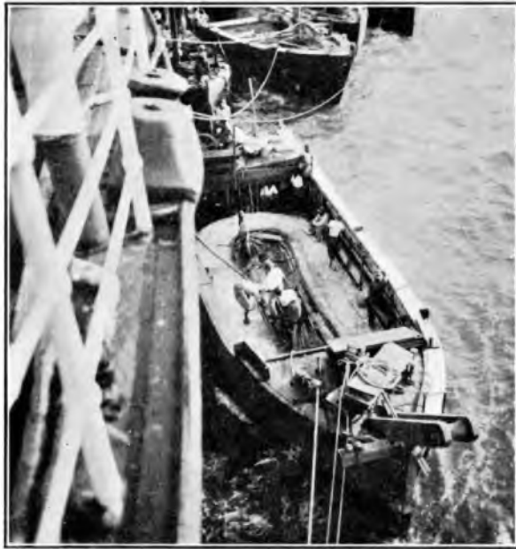
FIG. 3.—SHOWING THE CABLE IN THE LIGHTER.
