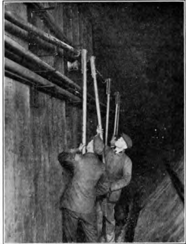
FIG. 9.—LOWERING CABLE TO FINAL POSITION.
