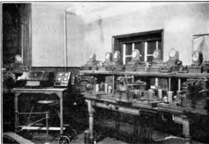
FIG. 1.—OLD TELEGRAPH REPEATER STATION, NEVIN.
