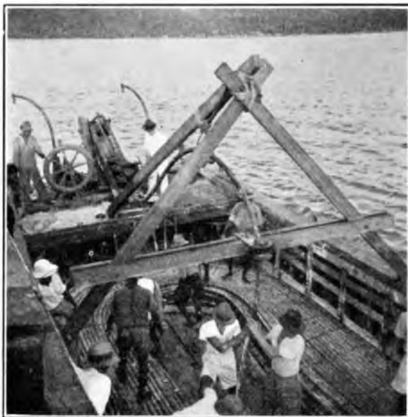
FIG. 4.—LAYING THE CABLE FROM THE LIGHTER.
