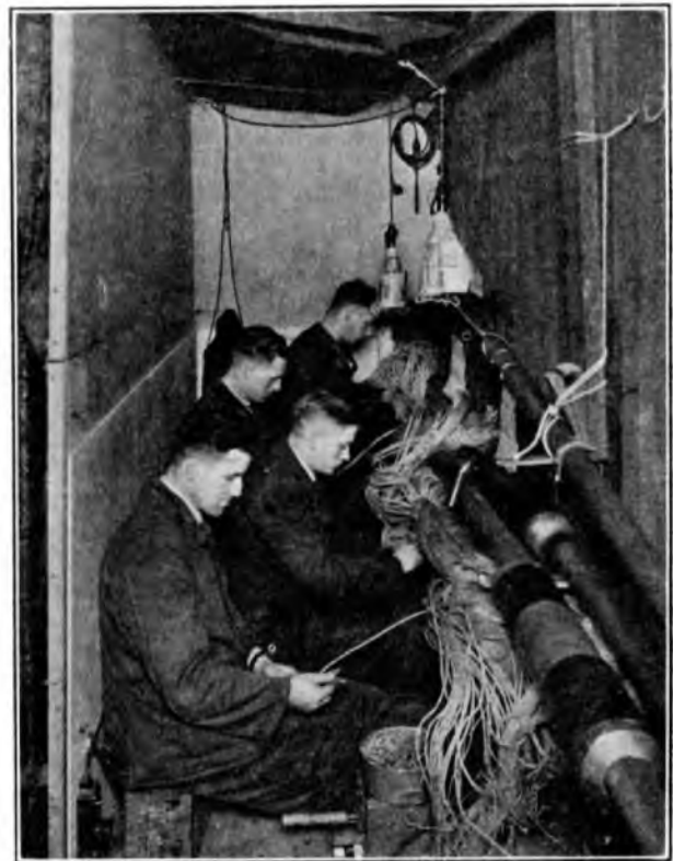
FIG. 11.—JOINTING WORK IN PROGRESS.
