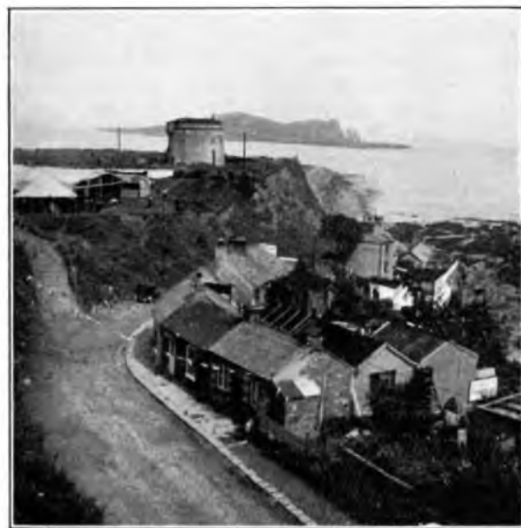
FIG. 4.—CARRIER REPEATER STATION AT HOWTH.
