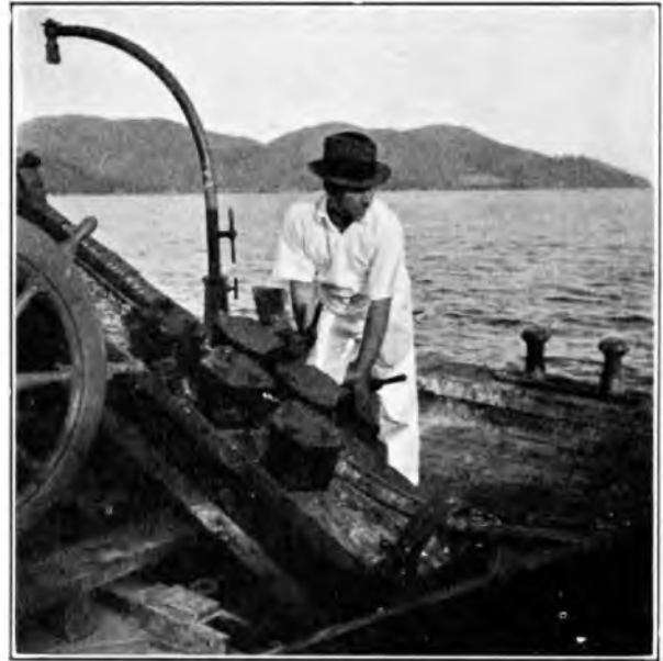
FIG. 7.—CABLE BRAKE IN OPERATION.
