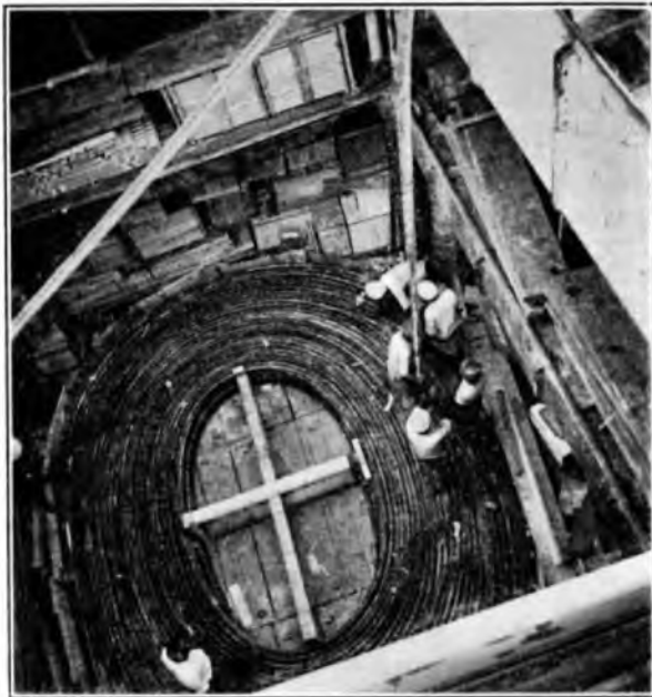
FIG. 1.—CABLE BEING UNLOADED FROM SHIP'S HOLD.
