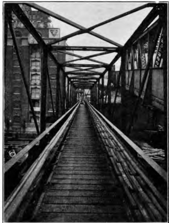
FIG. 4.—WARREN TYPE STEEL CABLE BRIDGE.
