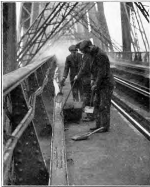
FIG. 4.—FILLING THE TROUGH WITH COMPOUND.
