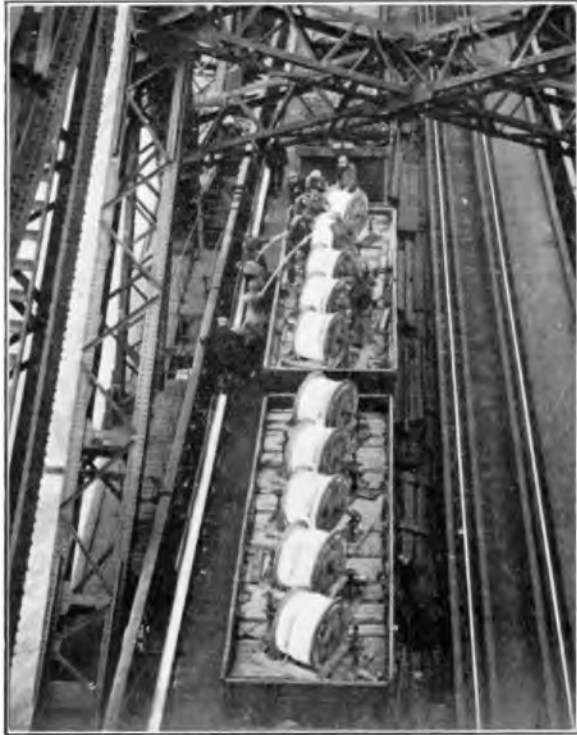
FIG. 6.—CABLE LAYING OPERATIONS.
