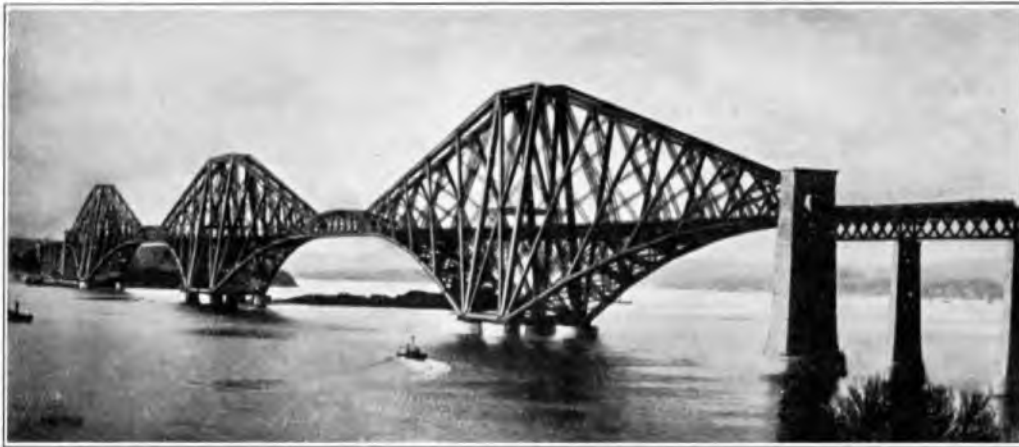
FIG. 1.—THE FORTH BRIDGE.
