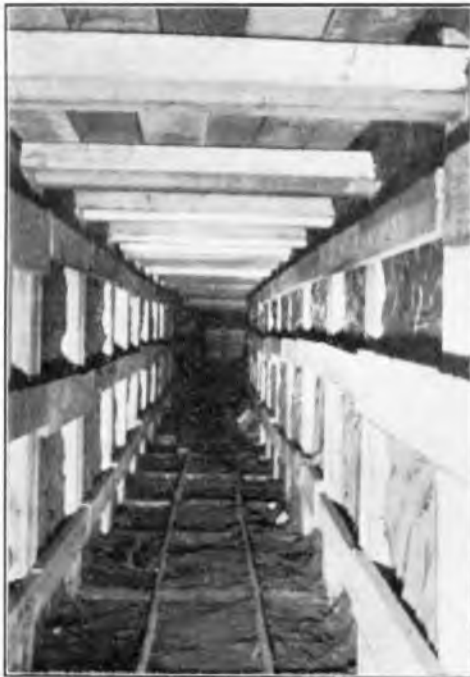
FIG. 1.—HEADING FOR 99-WAY DUCT ROUTE.
