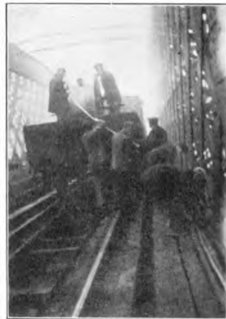
FIG. 2.—CABLE LAYING OPERATIONS.
