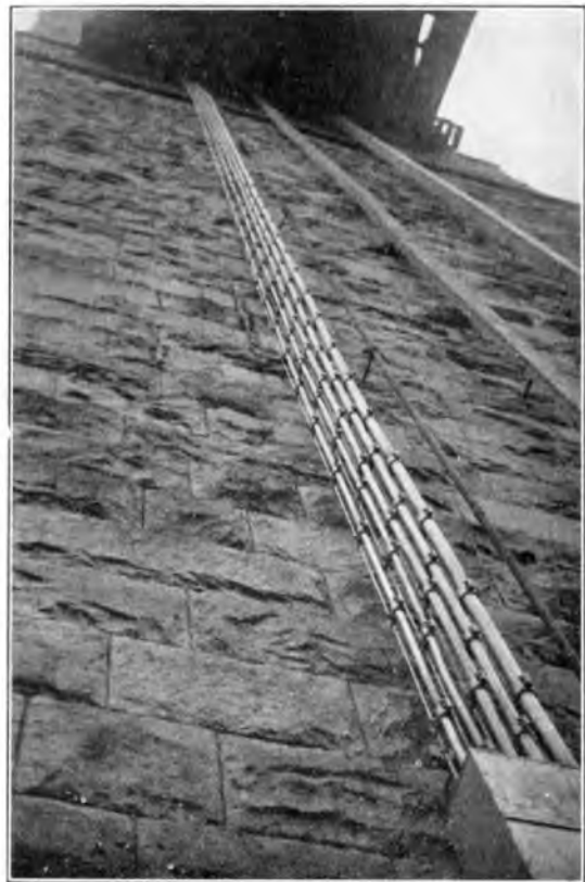
FIG. 5.—VERTICAL CABLE SUSPENSION ON NORTH PIER.
