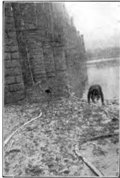
FIG. 4.—PAYING OUT THE WIDNES SHORE END.
