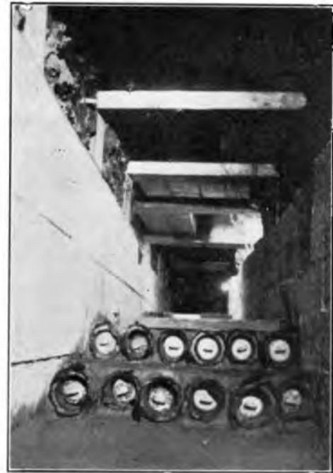
FIG. 2.—BOTTOM LAYERS OF 36-WAY DUCT ROUTE.
