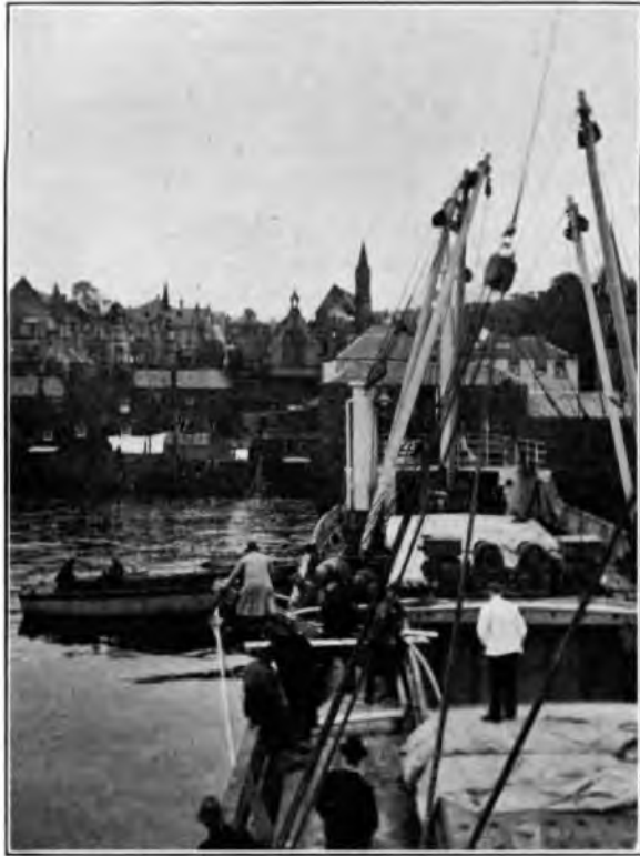
FIG. 2. PULLING THE SHORE-END OUT OF THE HOLD.
