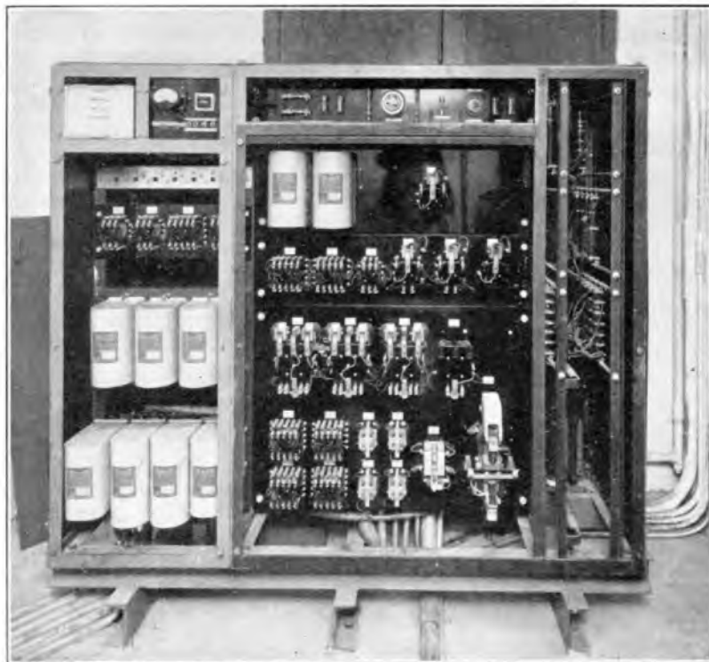
FIG. 2—FACE OF DUAL VOLTAGE CONTROLLER.
