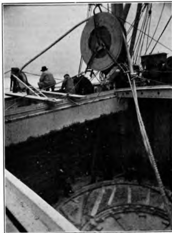
FIG. 1. PAYING OUT CABLE NO. 2 IN DEEP CHANNEL.
