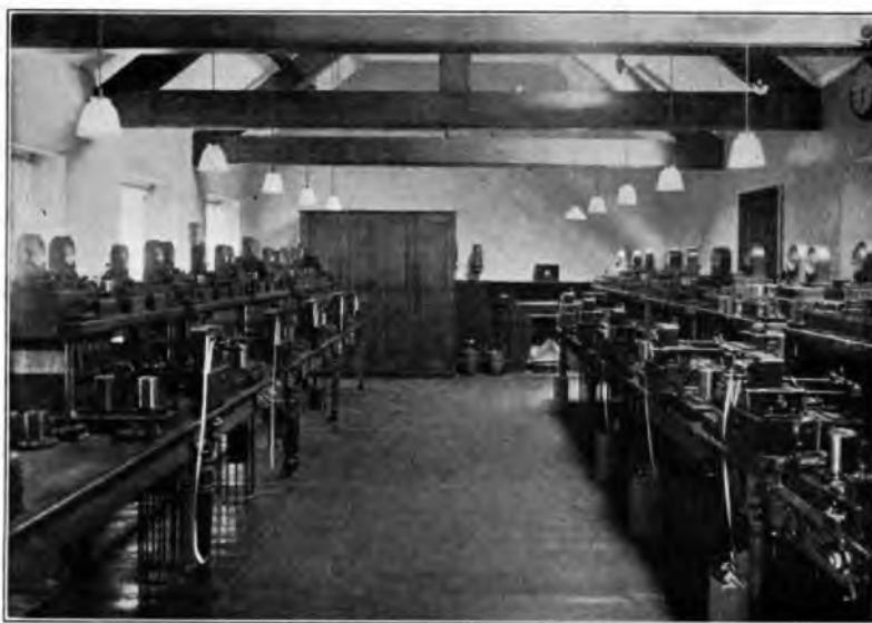
FIG. 2.—OLD REPEATERS AT THE LLANFAIR STATION.
