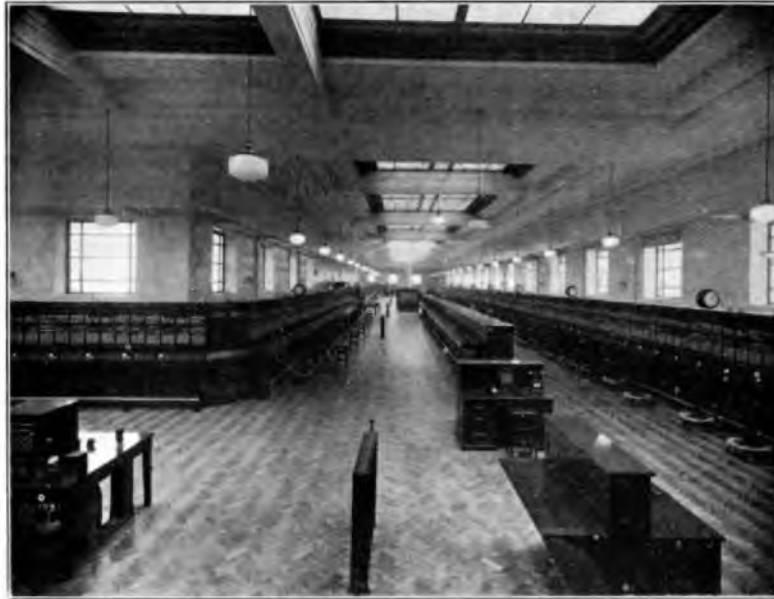
FIG. 3.—VIEW OF SWITCHROOM.
