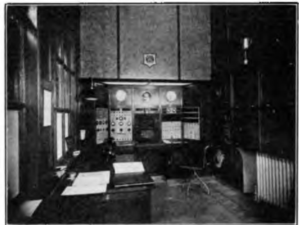
SWITCHBOARD IN THE WATCH ROOM.
