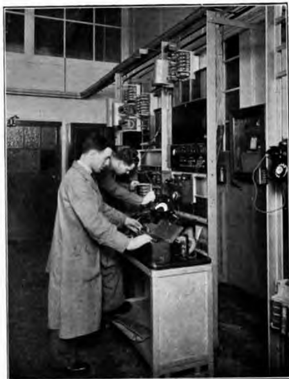
FIG. 3.—TESTING AUTOMATIC EQUIPMENT ON THE RACKS.
