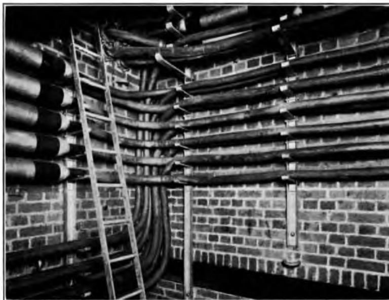
FIG. 5.—WEST WALL, LONDON WALL MANHOLE.
