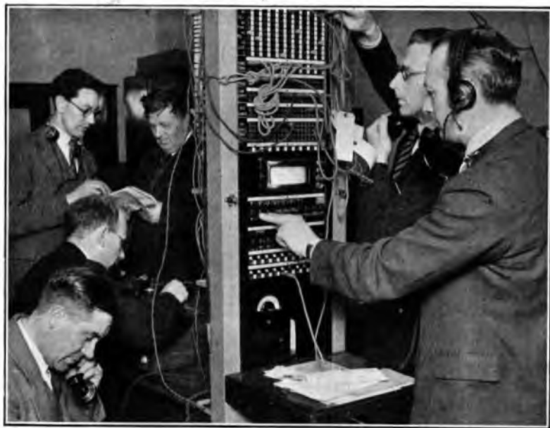
FIG. 1.—SETTING UP ADDITIONAL CIRCUITS AT KING'S LYNN.
