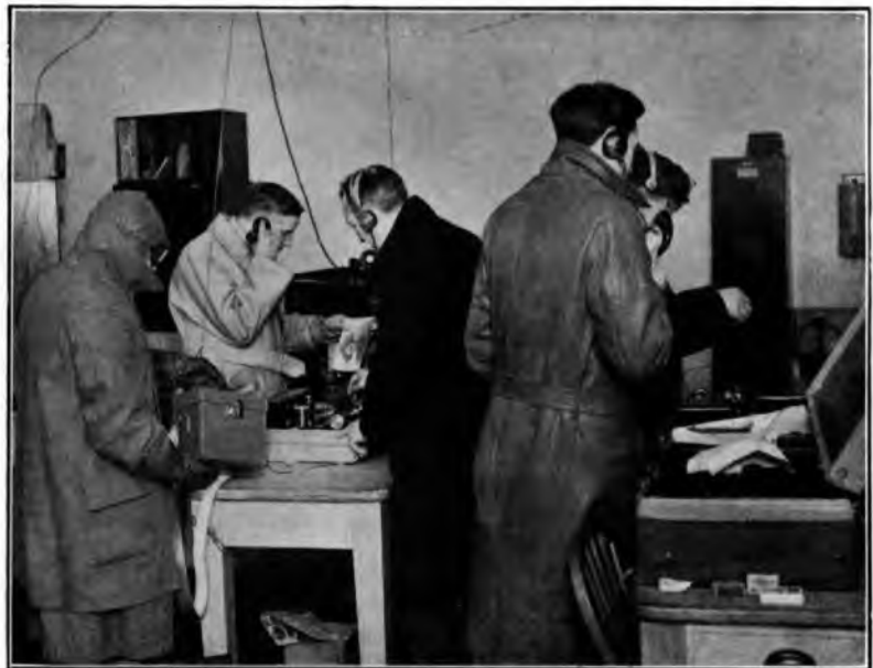
FIG. 5.—LINEMEN'S ROOM IN USE FOR PICTURE TRANSMISSION.
