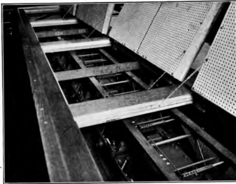
FIG. 11.—LETTER DISCHARGE MECHANISM.
