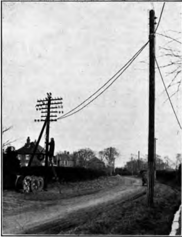
FIG. 2.—TEMPORARY CABLE BEING RUN.
