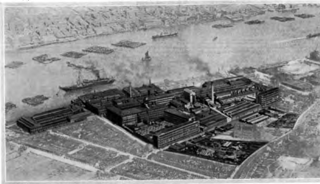
Aerial view of the Company's Woolwich Works and Cable Ship "Faraday." The River Thames in the background.
