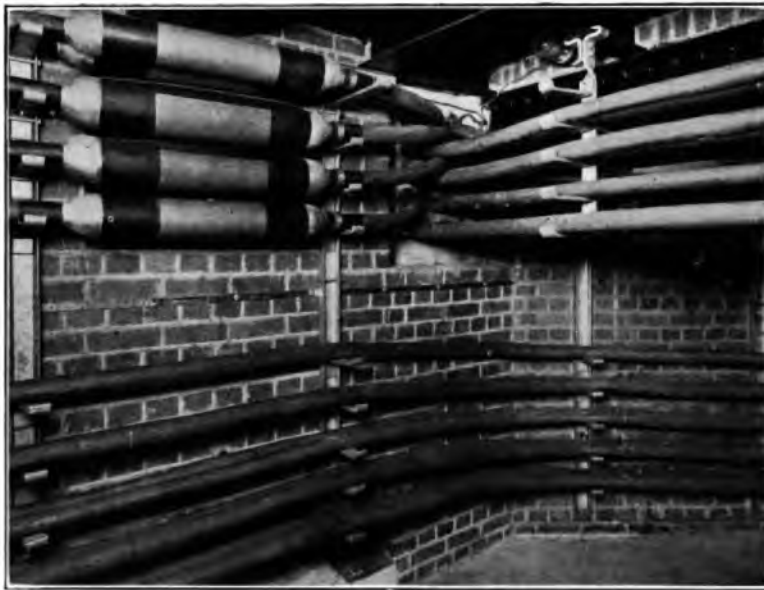
FIG. 6.—EAST AND SOUTH WALLS, LONDON WALL MANHOLE.
