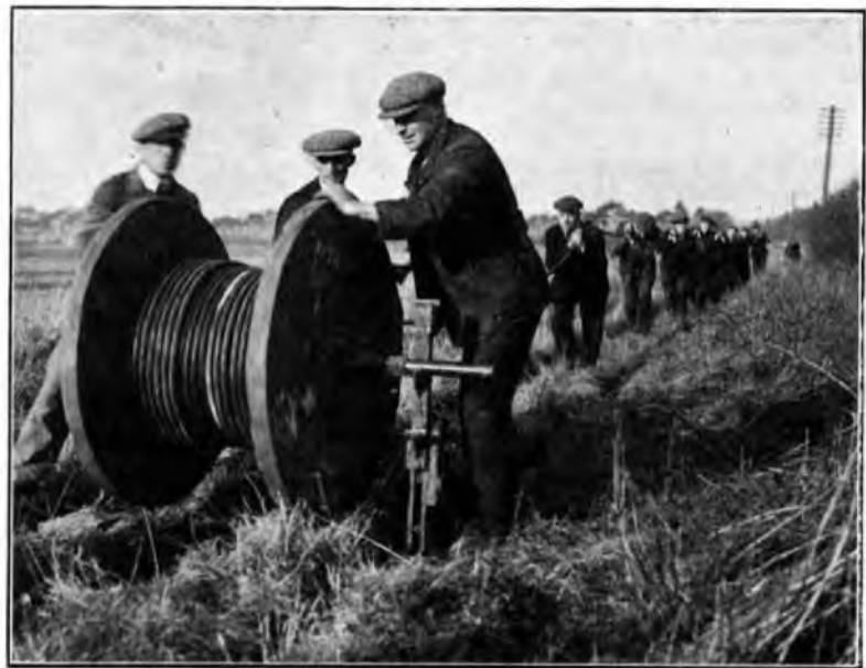
FIG. 3.—HAULING TEMPORARY CABLE BY HAND.
