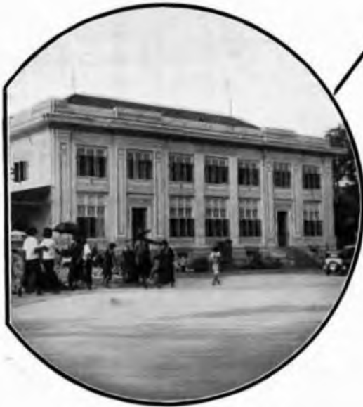
The Telephone Exchange building which will accommodate the automatic equipment serving the Wat Lieb area.
