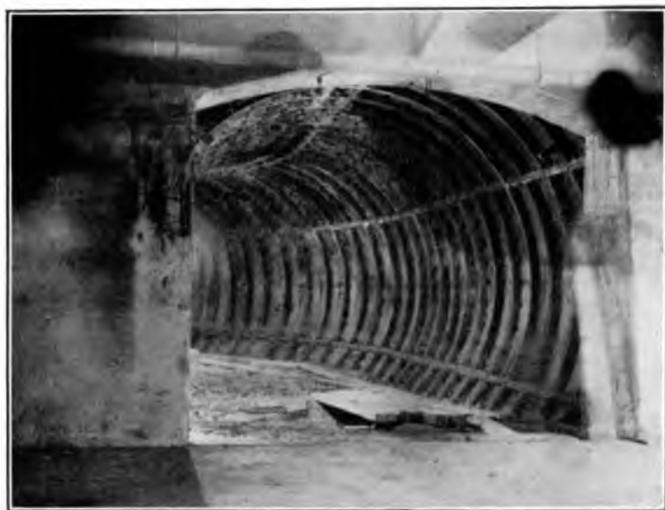
FIG. 2.—END OF TUNNEL IN COURSE OF CONSTRUCTION.
