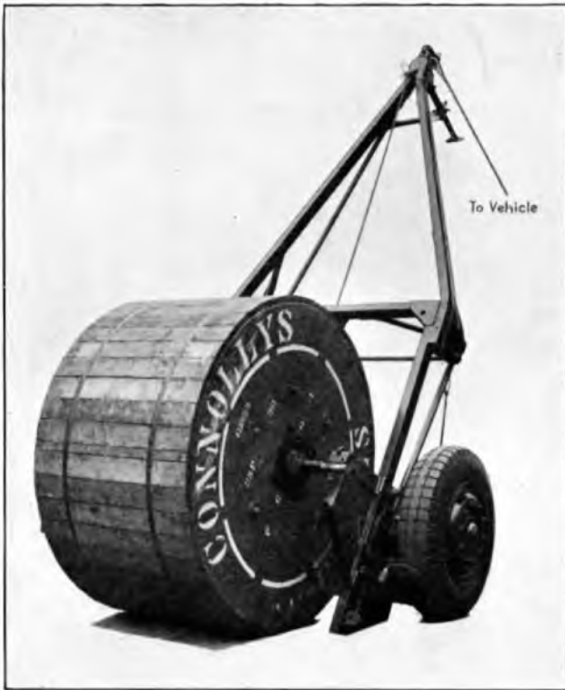
FIG. 2.—LOADING A 7' 0" DIAMETER CABLE DRUM.
