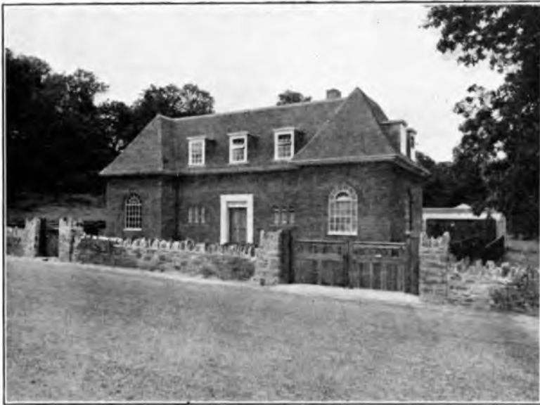
FIG. 5.—CROWNHILL SATELLITE EXCHANGE BUILDING.
