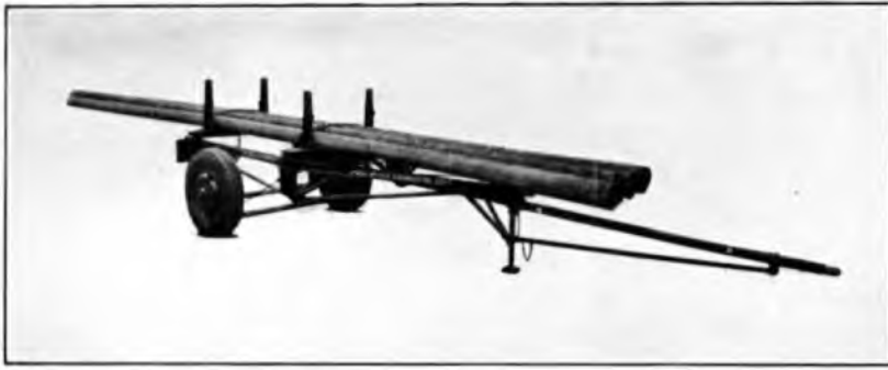
FIG. 4.—TRAILER EQUIPPED WITH BOLSTERS FOR CARRYING POLES.
