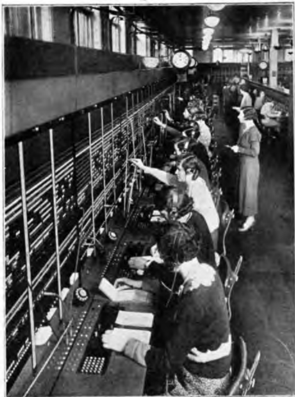
FIG. 9.—VIEW ALONG RADIO SUITE
