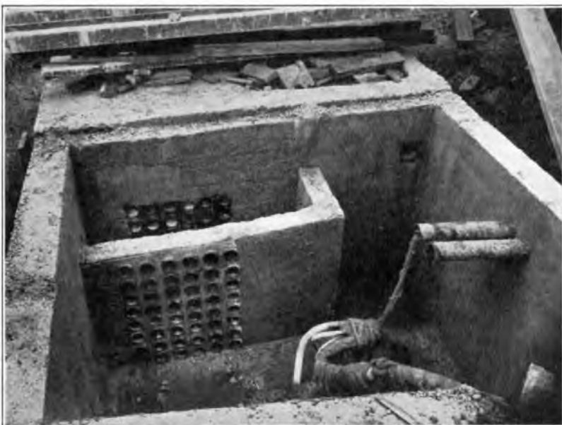
FIG. 2.—VIEW OF GREASE AND WATER CHAMBERS.
