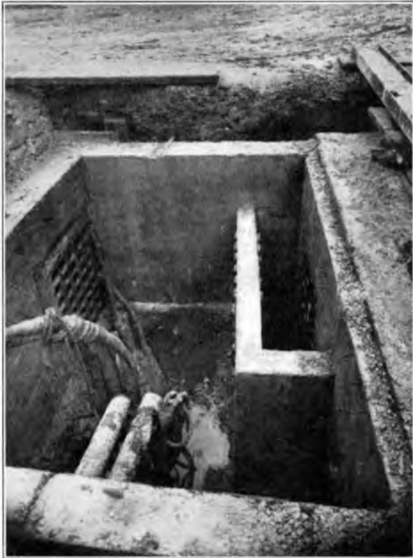
FIG. 3.—SIDE VIEW OF GREASE AND WATER CHAMBERS.
