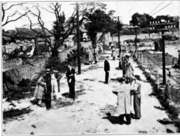
FIG. 2.—VIEW OF CONSTRUCTION PARK.
