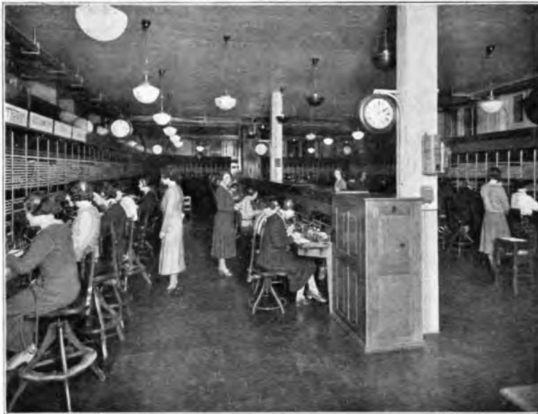
FIG. 4.—GENERAL VIEW OF SWITCHROOM.
