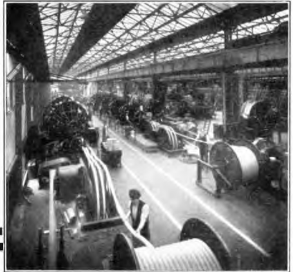
Laying-up Machines for Dry Core Cables.
