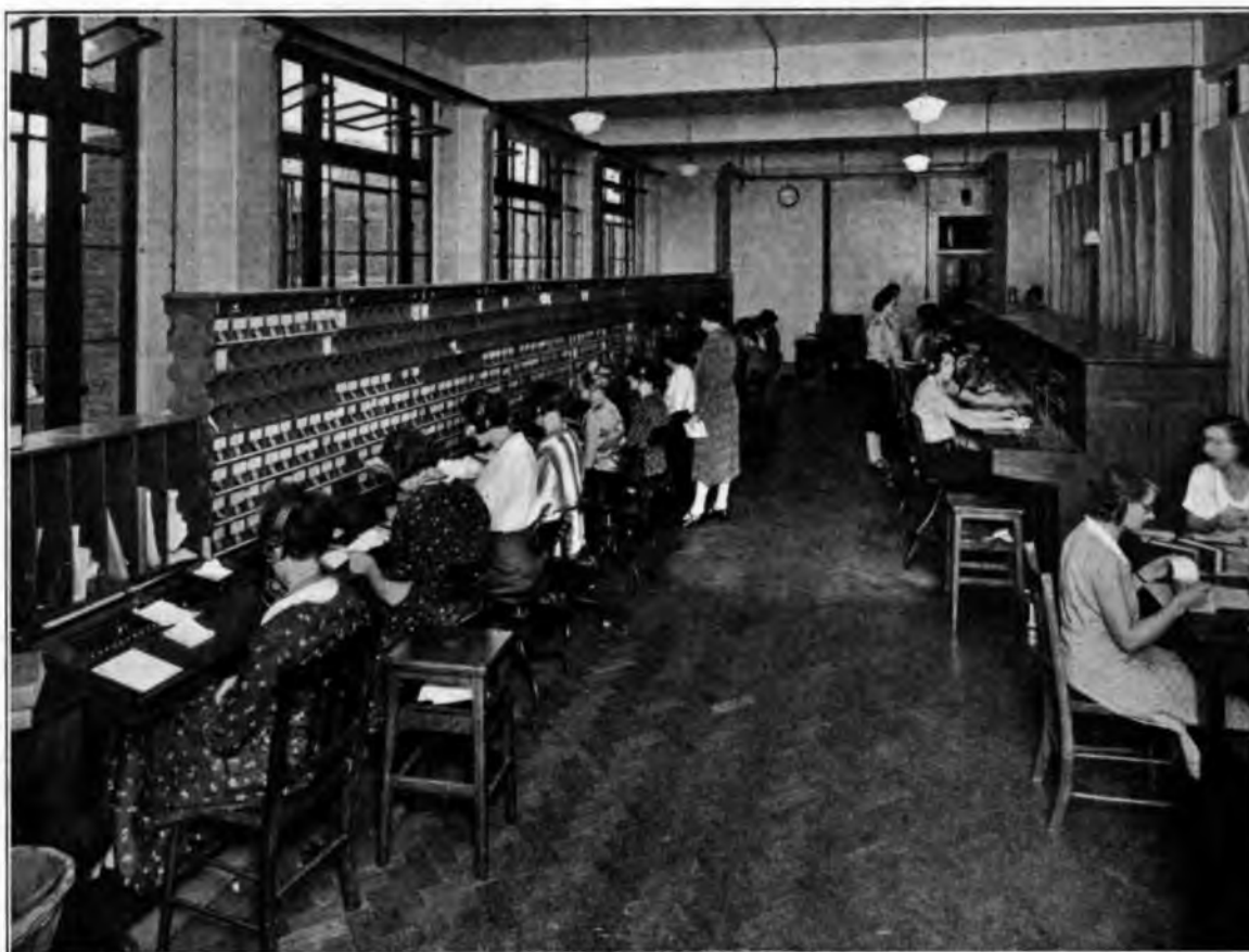
FIG. 1.—GENERAL VIEW OF SWITCHROOM.
