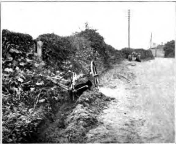
Fig. 9.—Plough drawn by winch with Furrow 10"—12" deep.
