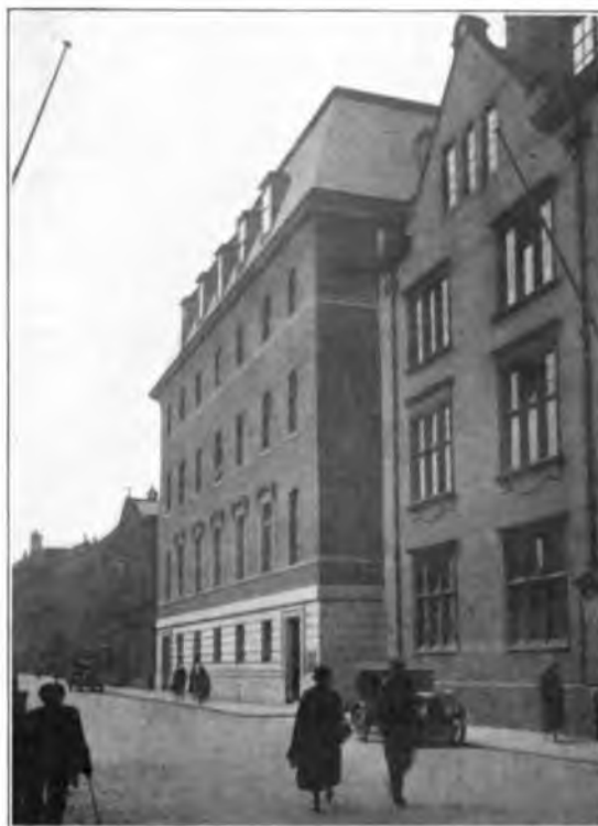
FIG. 2.—SUNDERLAND EXCHANGE BUILDING.
