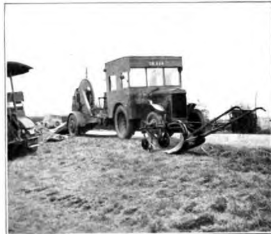
Fig. 12.—Rushton Tractor, Cable Bogey and Ransome Ridging Plough.
