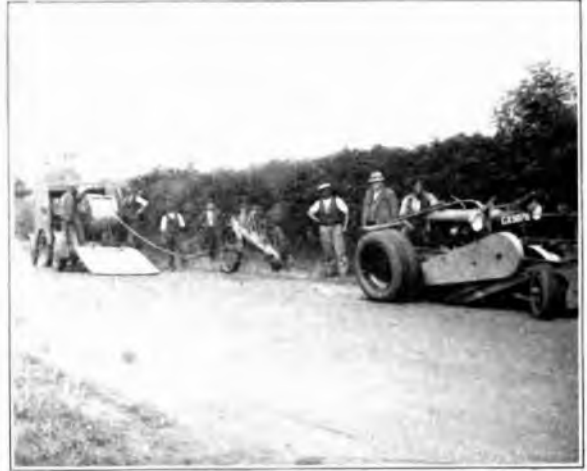
Fig. 6.—Tractor, Mole Drainer and Cable Bogey. Notice anchor and winding drum.
