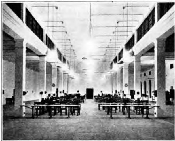
FIG. 5.—CENTRAL TELEGRAPH OFFICE, NEW DELHI. Photo taken at night. Shows arrangement of lights, fans and tables.
