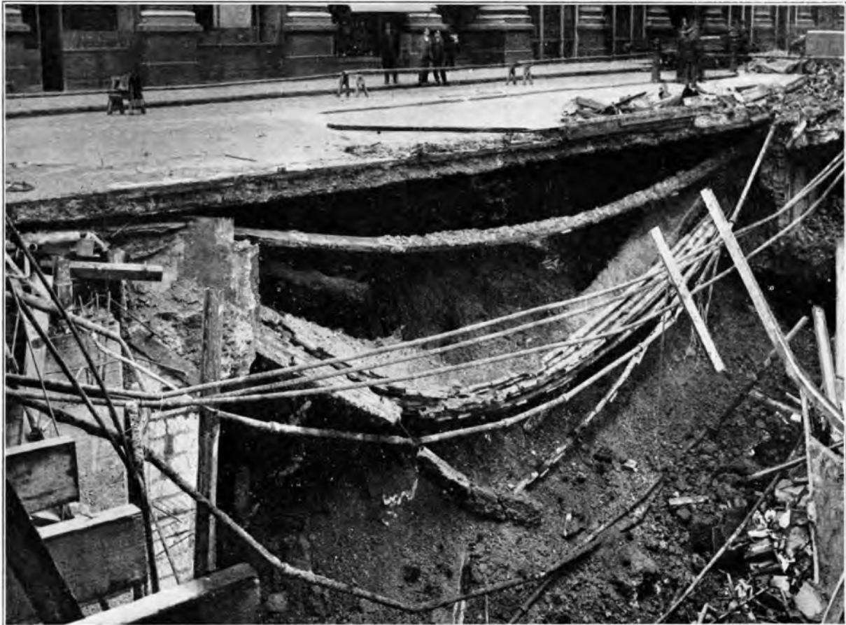
FIG. 2.—POST OFFICE MAIN DUCT ROUTE BENEATH ROADWAY AFTER SUBSIDENCE.
