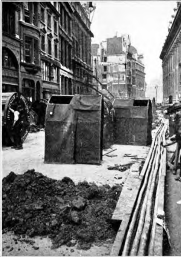
FIG. 3.—OPERATIONS IN CORNHILL SHOWING CABLES IN TROUGHING.
