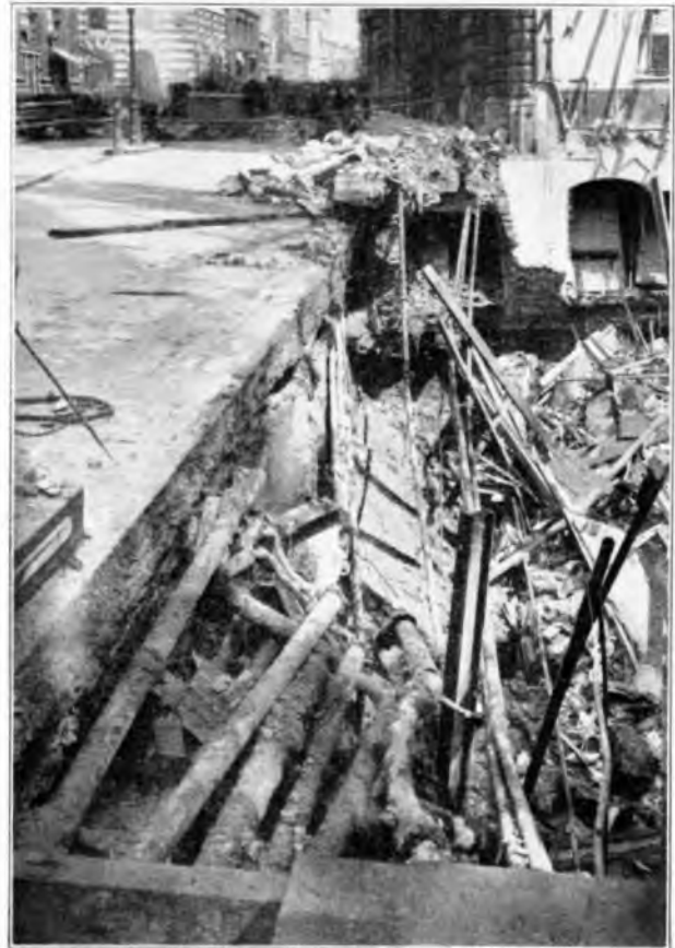
FIG. 1.—SITE IMMEDIATELY AFTER COLLAPSE OF BUILDING.
