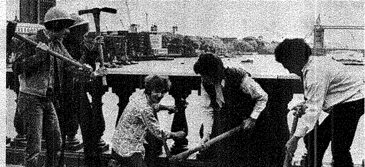
The SPECTRUM, lending a helping hand demolishing London Bridge. (l to r) ANTHONY JUDD, KEITH and COLIN FORSEY, TONY ATKINS and BILL CHAMBERS.
