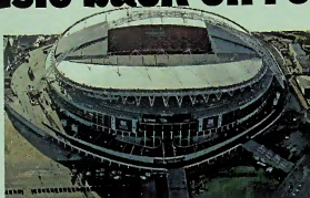
Underneath the arches: feedback about the new Wembley has been positive
