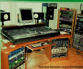
Technical Services: recent installation
