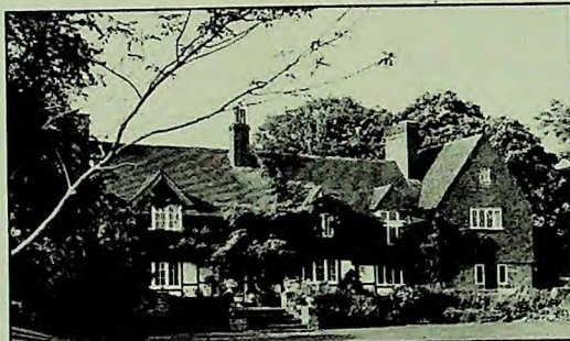
THE MAIN House at Stanbridge
