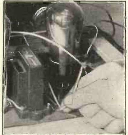
Every connection should be mechanically sound. When a receiver suddenly develops a background crackle, go over all the joints and make quite sure that they are tight.
