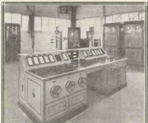
The white rectangles on the control desk looking like writing pads are actually drum-dialled meters.
