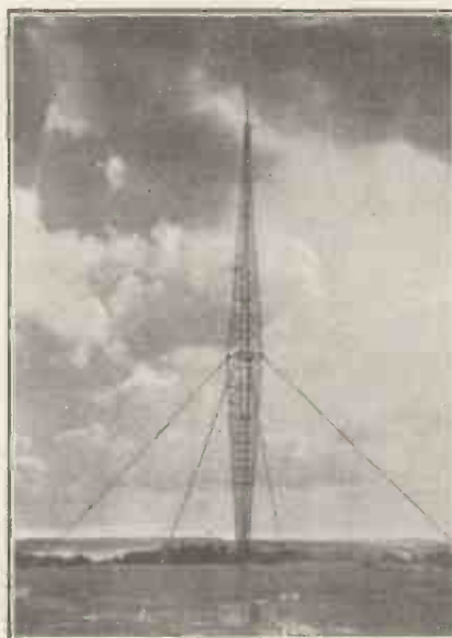
A vertical aerial is used at the Newton Square station, and it is supported inside this peculiarly-shaped wooden mast. It is 500 feet high.
