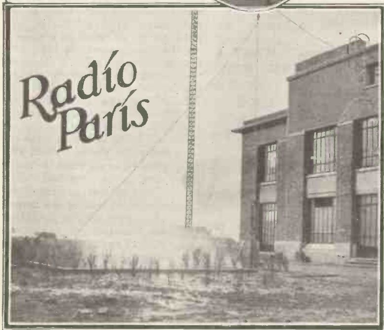
Radio Paris transmits on 1,725 metres, with a power of 75 kilowatts. This exterior view of the station shows the main lead-in—or rather lead-out; whilst to the right is the grand staircase by which visitors enter the transmitting rooms.
