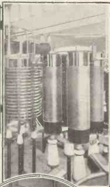
Above and to the right are close-ups in the transmitting-room, showing the elaborate insulation and adequate spacing necessary to handle the 12,000 volts high tension.
