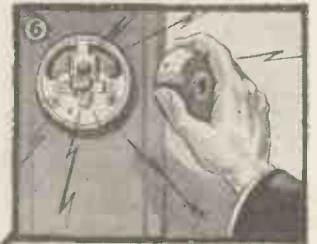
An ordinary wall switch for the lights is sparking.
