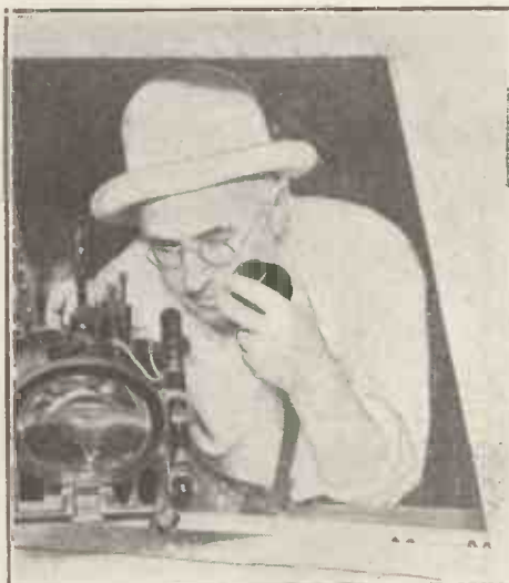
Mr. John Bellamy Taylor, of Schenectady, doesn't think much of wireless. He has just perfected the apparatus seen here which will send human speech on a beam of light. His invention opens up great possibilities for secret communication between aeroplanes and the ground, or ships and the shore.
