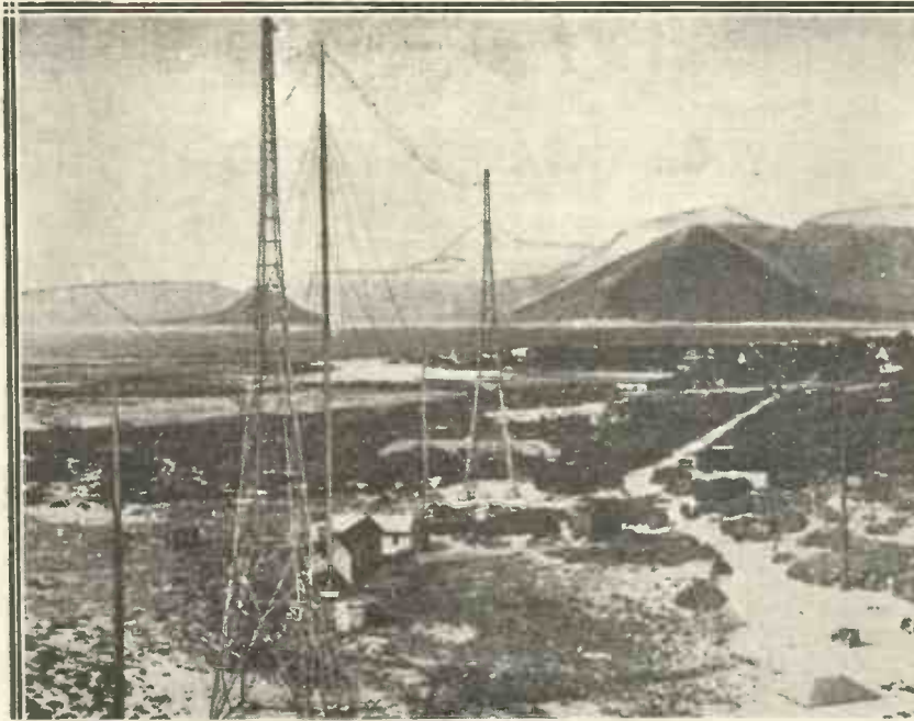
Situated on the Cape of Good Hope, about 50 miles from Cape Town, the famous Slangkop radio station keeps South Africa in touch with the great liners on the Atlantic and Indian Oceans. The towers shown have just been erected to replace the masts.
