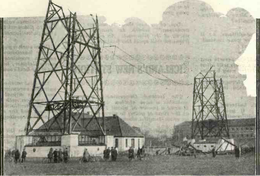
The famous wooden masts of Munich failed to withstand the recent winter gales and came down with a run one night. Fortunately, no one was injured, and the temporary aerial shown enabled the station to carry on as usual with its programmes on 533 metres.
