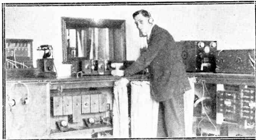
A corner of the control room at the Leeds-Bradford relay station. The future of such stations is still undecided, and is dependent upon the success or otherwise of the Regional Scheme.
