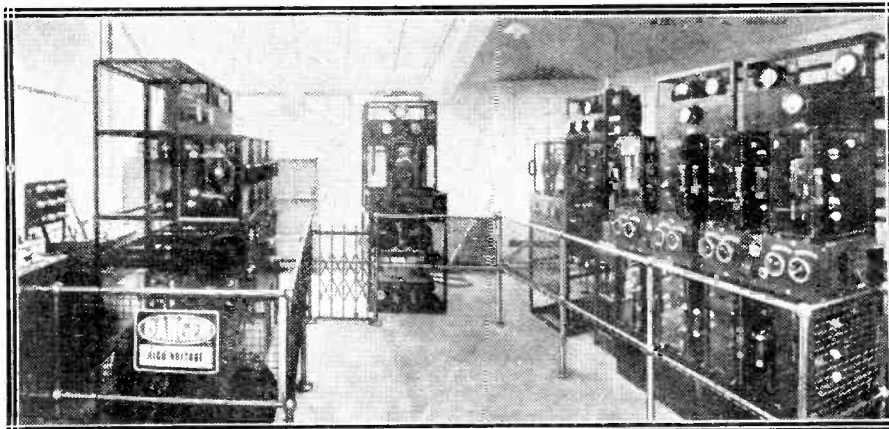
When the London station 2 LO was moved from the Strand to Oxford Street many alterations were made, and the transmitter was brought right up-to-date. This photograph shows part of the main transmitter, situated just beneath the aerial on the roof of Selfridges.
