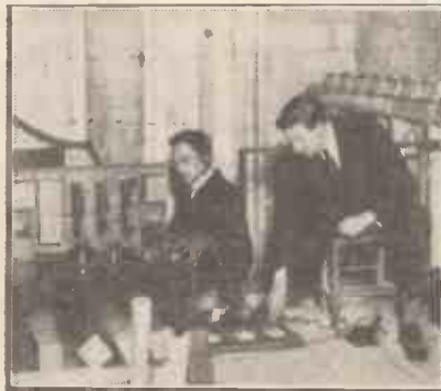
B.B.C. engineers installing a microphone in Canterbury Cathedral.
