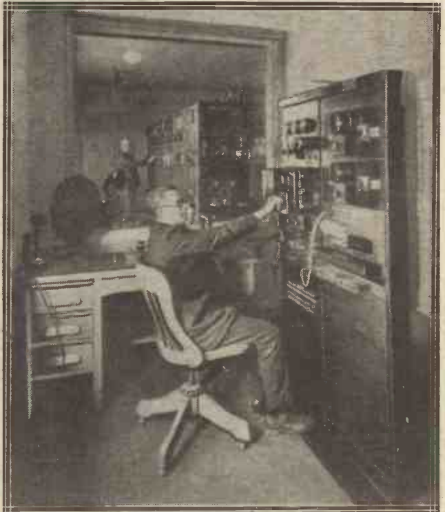
This is the control panel in the transmitting room. An unusual view of the transmitter itself is given through the large window in the background. This window has the appearance of a mirror, at least it has in the photograph, as will be noticed.
