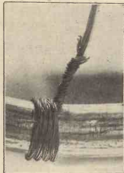
A bad method of making contact, which will corrode and cause trouble before long.
