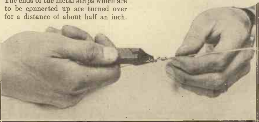
Pliers should gently, but firmly, be used for twisting wires together.
