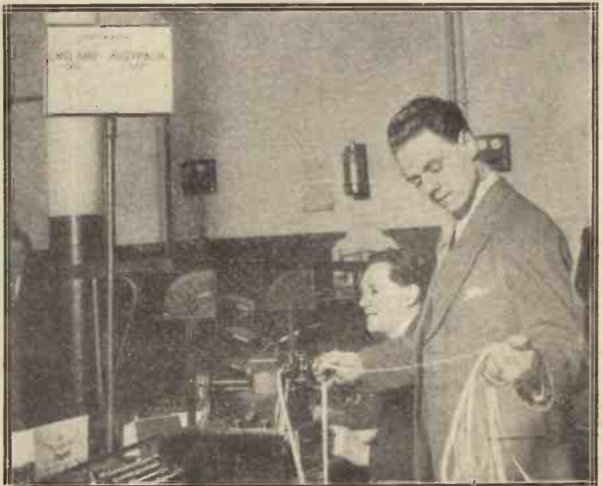
The apparatus in the Central Telegraph Office, London, which is used to transmit messages via the Beam to Australia.
