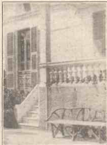
The author's house, showing the aerial lead-in.
