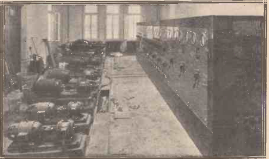
The generator room with its huge "panel" and controls.
