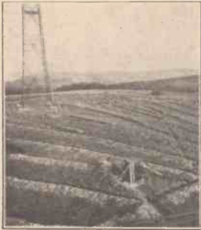
Some of the trenches in which the earth-wires are buried.
