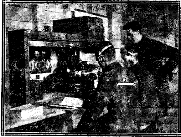
The training of Army wireless operators is carried out on up-to-date valve apparatus
