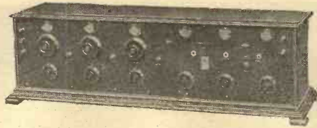
THE ANGLO-AMERICAN SIX. Mr. Percy Harris' latest Set embodying three stages of neutrodyne high-frequency. Gives practically the power of a super-heterodyne with a great saving in valves. A few feet of wire around the picture moulding of a room is all that is necessary to operate this Set.
