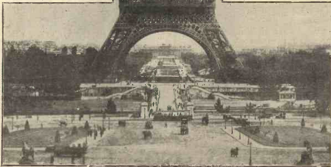
A view of the famous Eiffel Tower, Paris, which is used for supporting the aerial of the wireless station, a description of which appears in this article.
