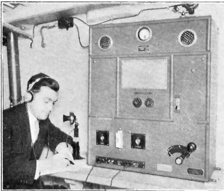
The Marconi telephone equipment installed in the new Dover lifeboat.
